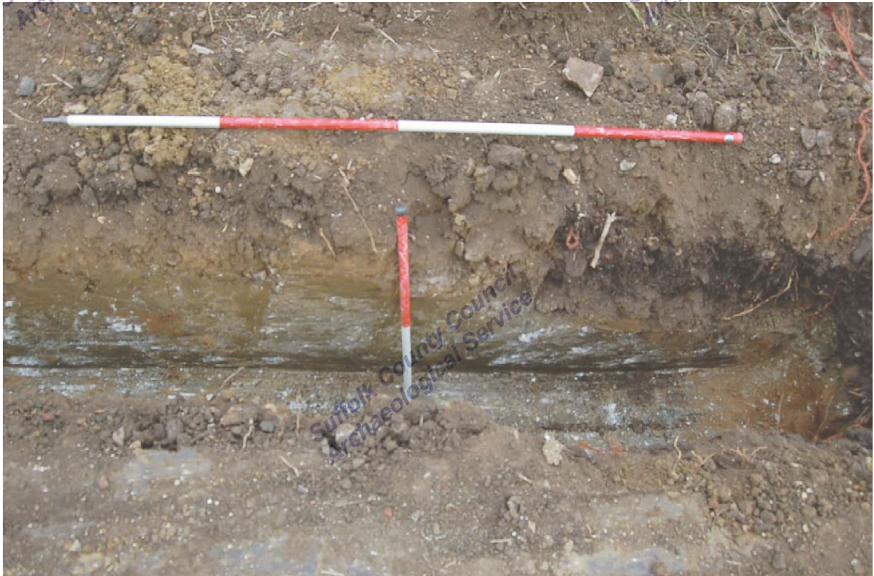
Plate 2. Detail of modern disturbance at southern corner of garage foundations, facing south.
