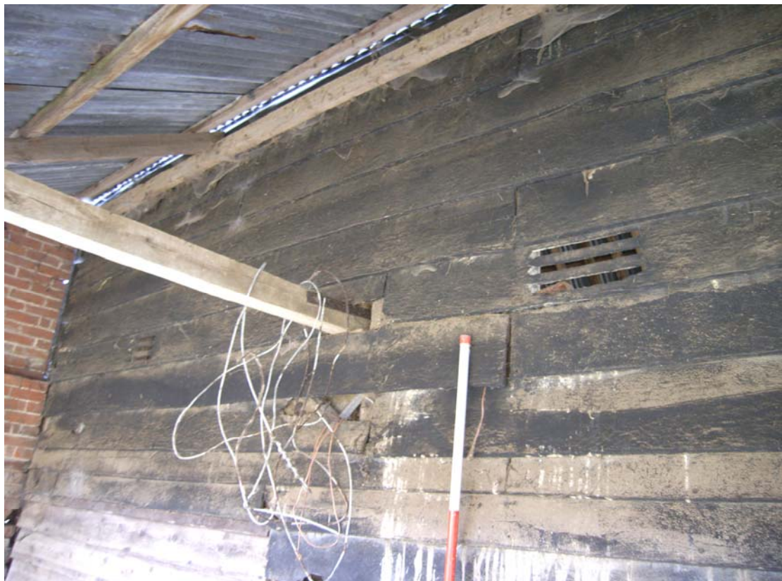
A2.4 Unusual horizontal ventilation slits in tarred external northern weatherboarding of 19 th century barn (3) seen from lean-to shelter shed (5).
