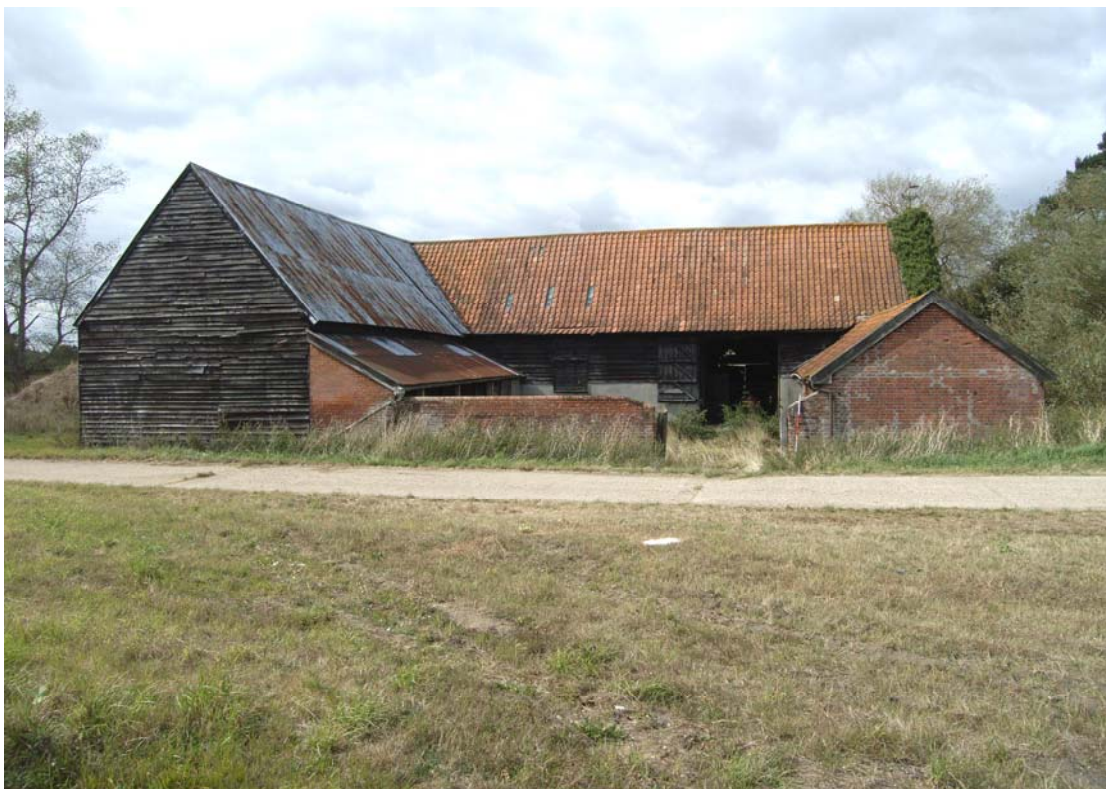
A2.2 Exterior of complex from east showing 19th century yard entrance in foreground, 19 th century barn (3) to left and 16 th century stable range later converted into a barn (1) in rear
