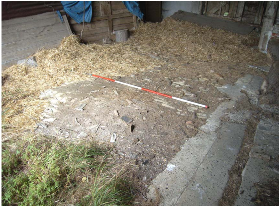
A2.6 Threshing floor of white brick in central bay of 19 th century barn (3), viewed from southern entrance.
