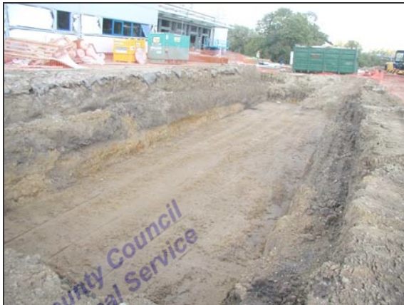
Plate I: general view of storm water tank excavation looking northeast (7 th Oct 2004)
