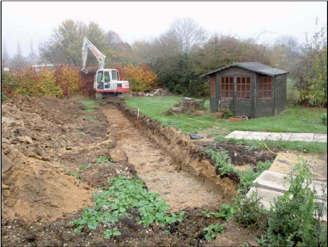
Plate I. General view of Trench 1 looking north (ref. GER 54)
