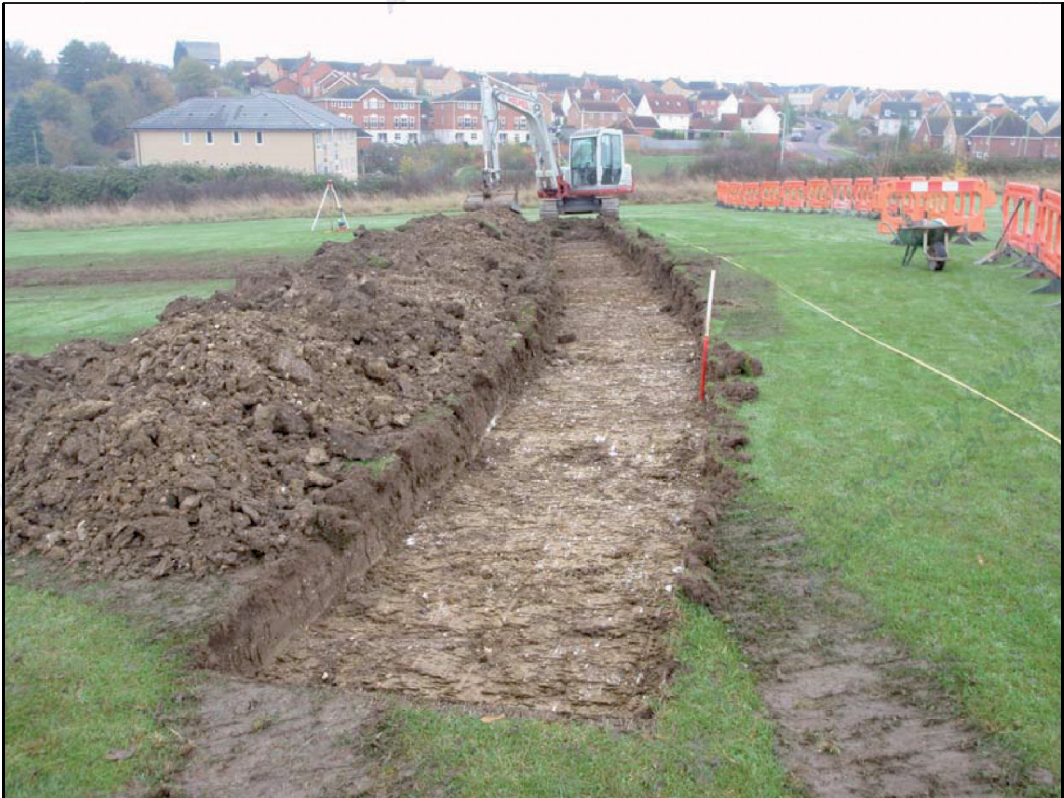
Plate II. General view of Trench 2 looking south (ref. GER 60)
