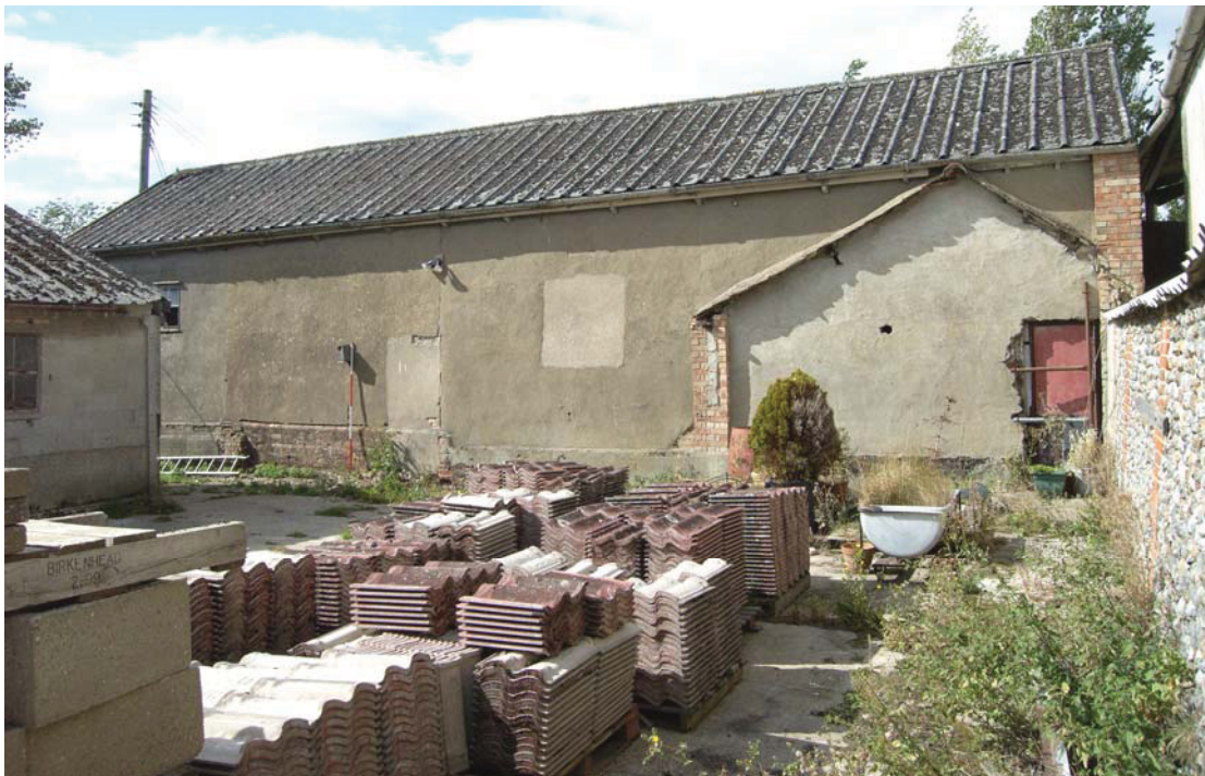
A2.2 Southern exterior of the cement-rendered barn showing the mid-20 th century cow shed to left and the roof scar of the demolished 19 th century shelter to right. The blocked original entrance is indicated by a section of darker render to the left
