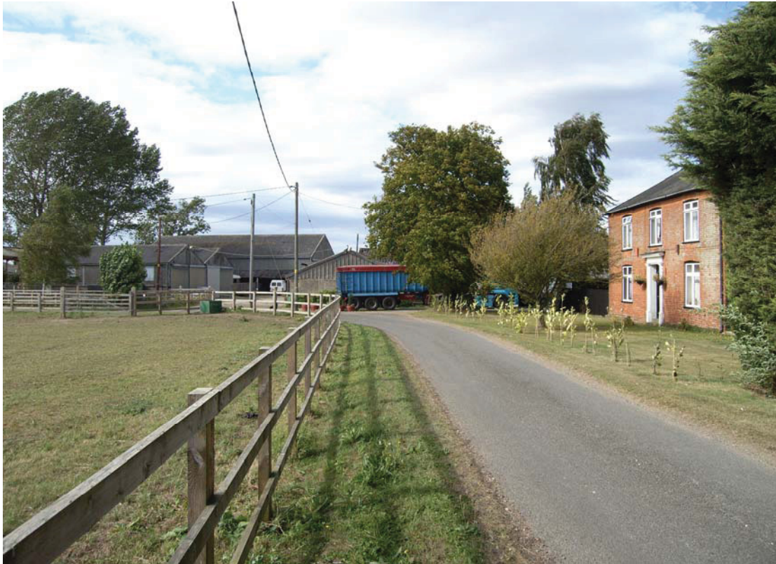
A2.1 General view of site from Church Lane to south showing mid-19 th century farmhouse to right. The roof of the historic barn is just visible above the blue truck, with 20 th century sheds to the left
