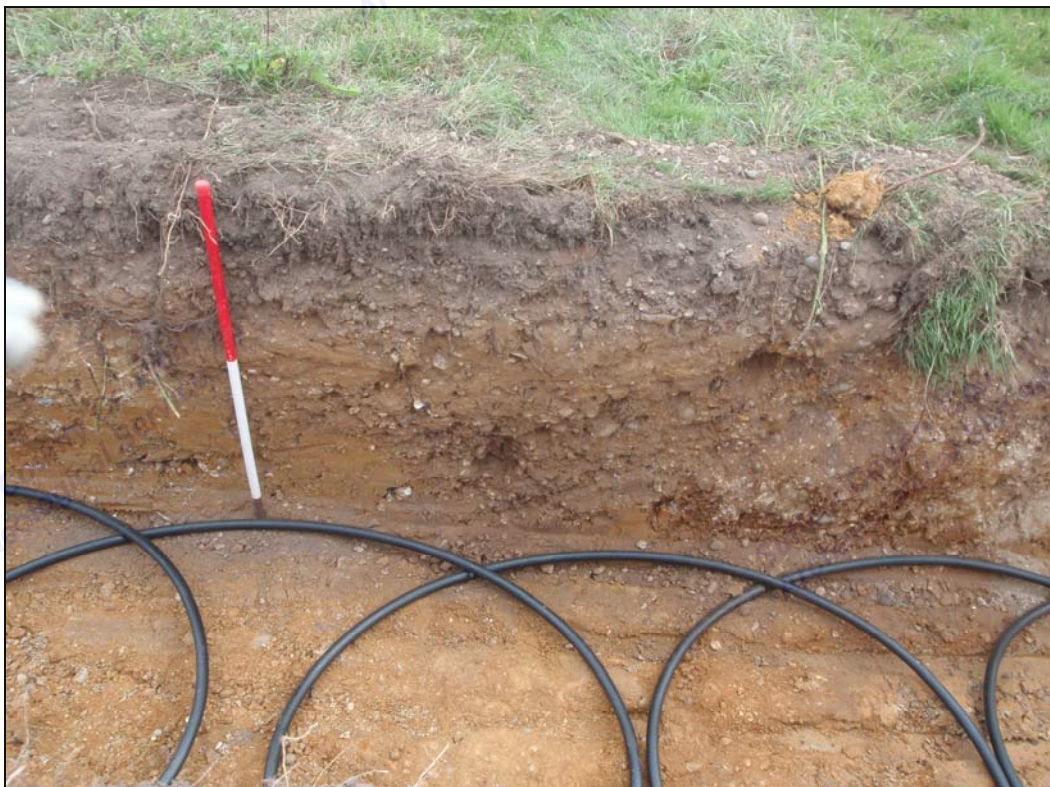
Plate II. View of ditch 0004 in northern ground source heating trench, looking SE (1m scale, photo ref. GET 48)
