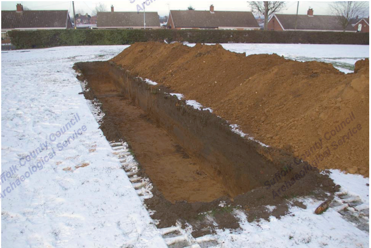
Figure 4. General view of Trench 4, looking north
