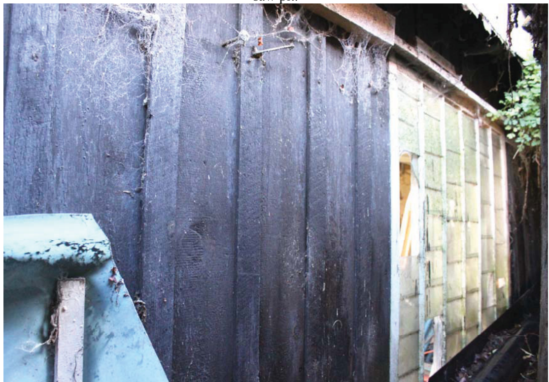
A2.9 Shed 1. Detail of original tarred external northern cladding showing vertical boards with fillets concealing abutments (seen from shed 2).
