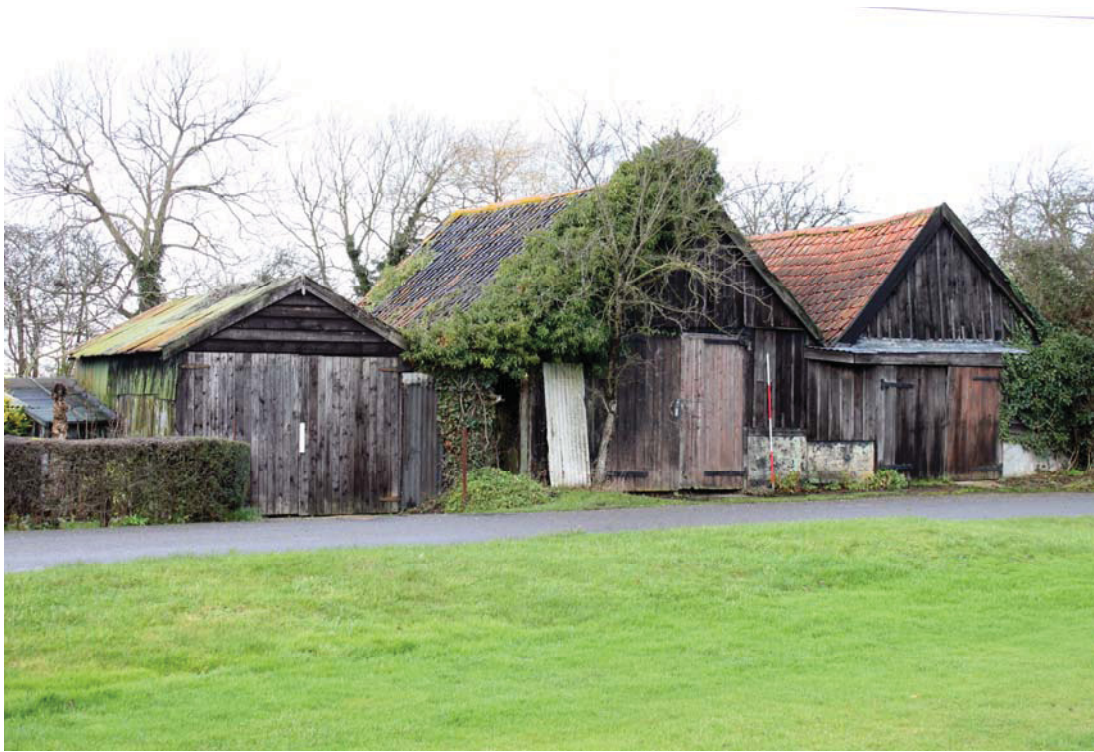
A2.2 Exterior from south-east showing the black glazed pantiles of shed 1 to left and the red pantiles of the later shed 2 to the right. The smaller shed to the extreme left is the garage of the neighbouring property (Holly Cottage)
