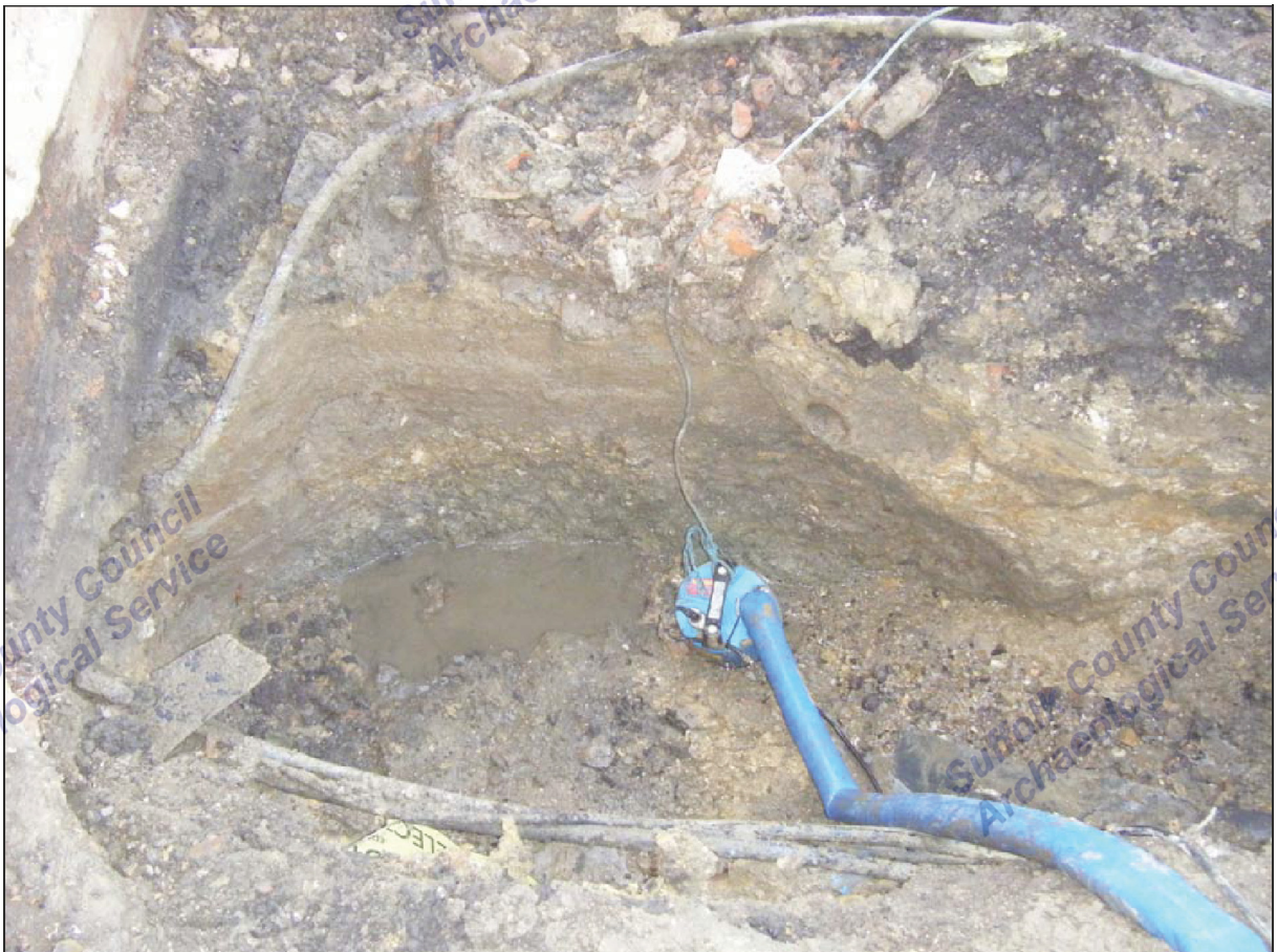
Plate 1. Soakaway in extension foundation trench showing ceramic pipe, looking south
