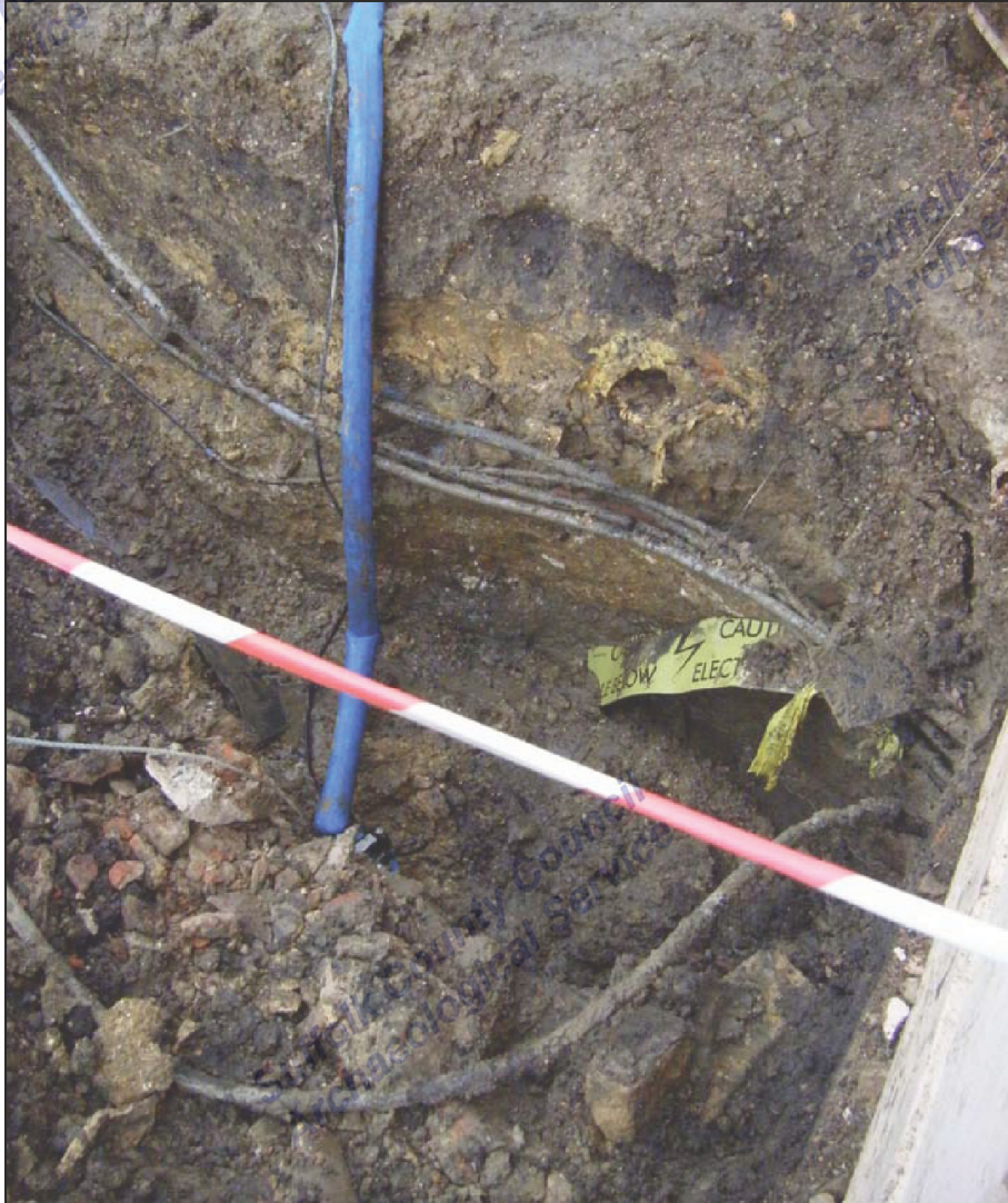
Plate 2. Service trench running into soakaway in extension foundation trench, looking north-west
