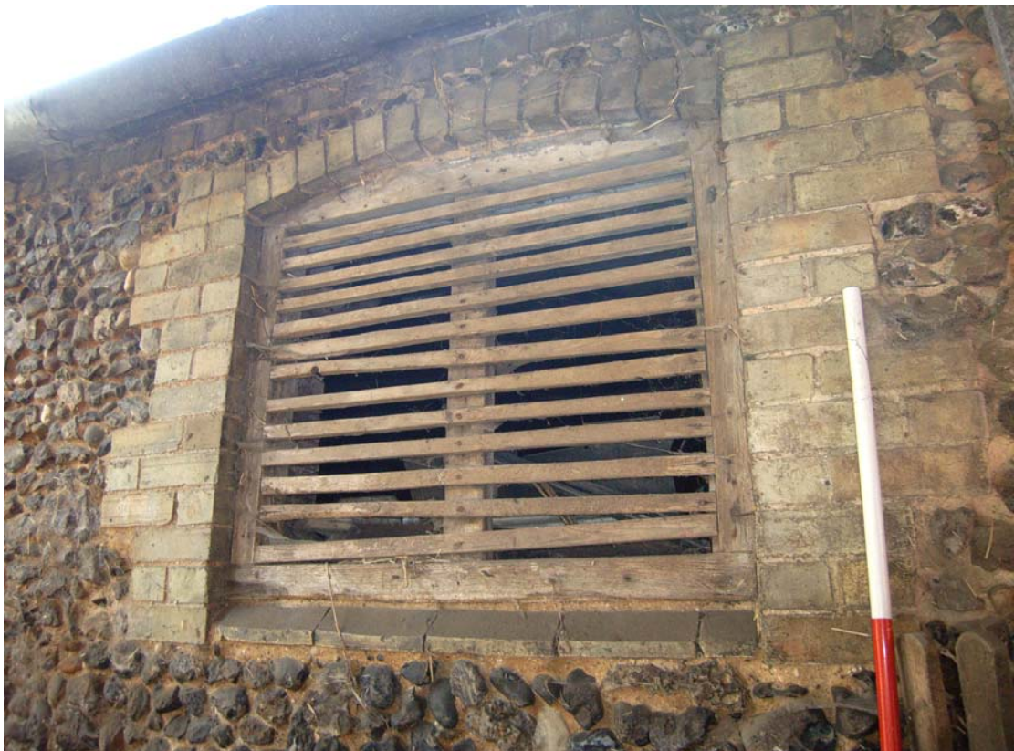
A2.10 Stable (8). Detail of northern louvered window in western exterior.
