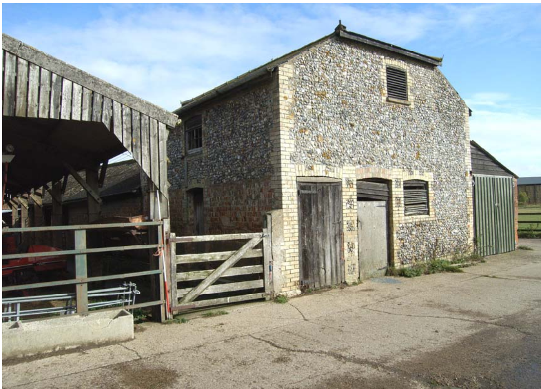
A2.8 Granary (6). Exterior from south-west showing 20th century covered yard to left. The left-hand door of the southern gable opens onto an original internal stair.
