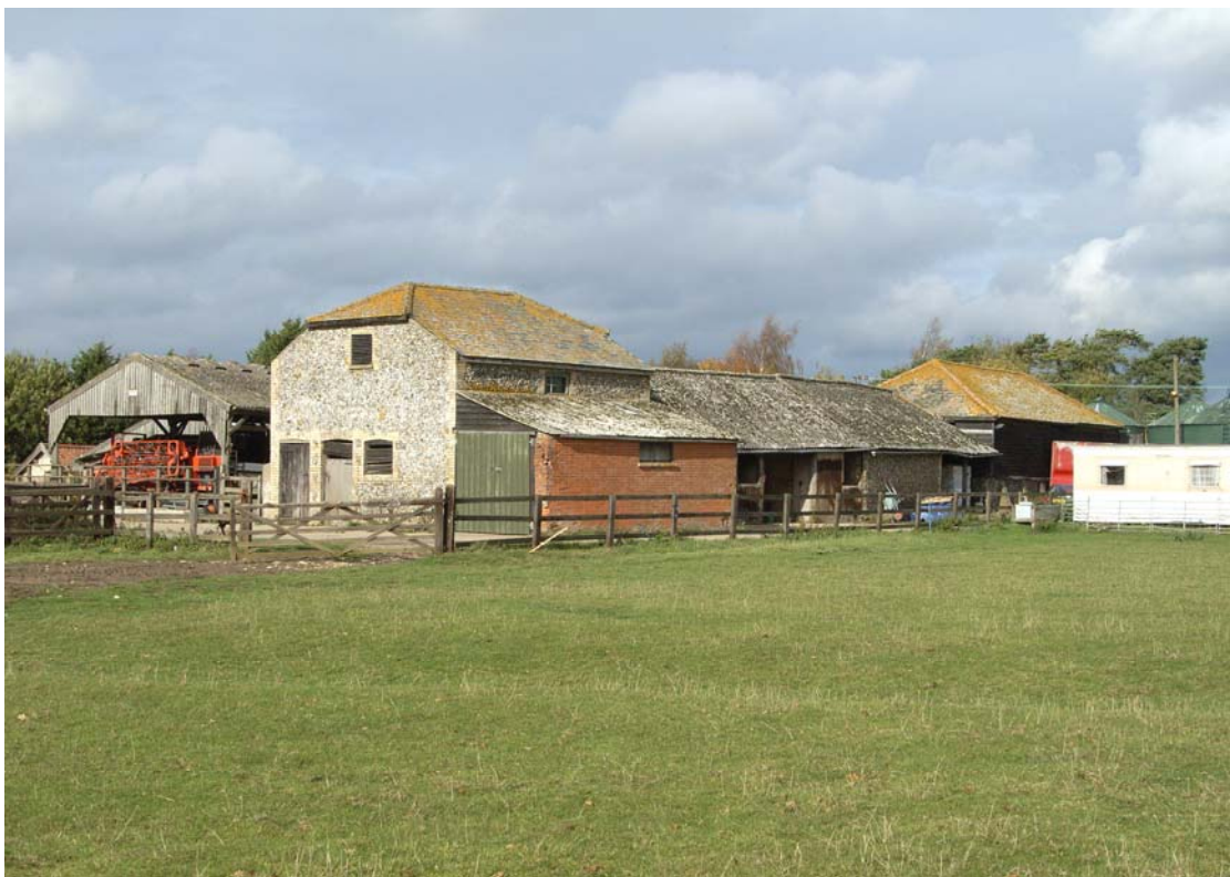
A2.2 General view of site from south-east showing granary (6) to left and barn (3) right
