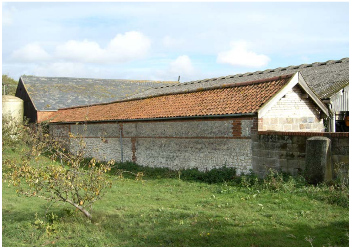
A2.12 Shelter shed (9). Exterior from south-west showing clunch construction with brick dressing and slate roof of western barn (1) to left.
