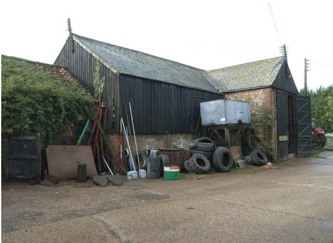
A2.4 Western Barn (1). Exterior from north-east showing slate roof with northern porch and tall plinth of clunch and flint rubble. The vehicle shed (2) is visible to the left
