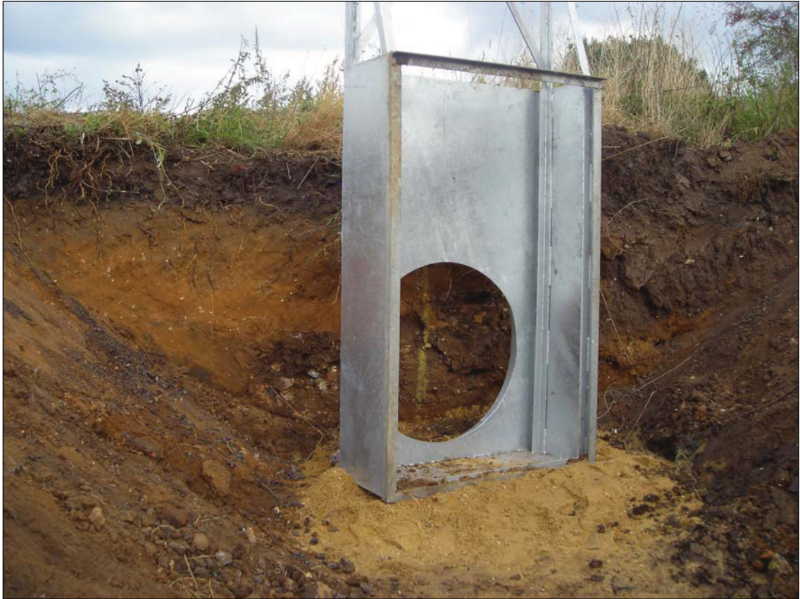
Plate 3. Sluice gate excavation showing NW-SE section drawn as Figure 3
