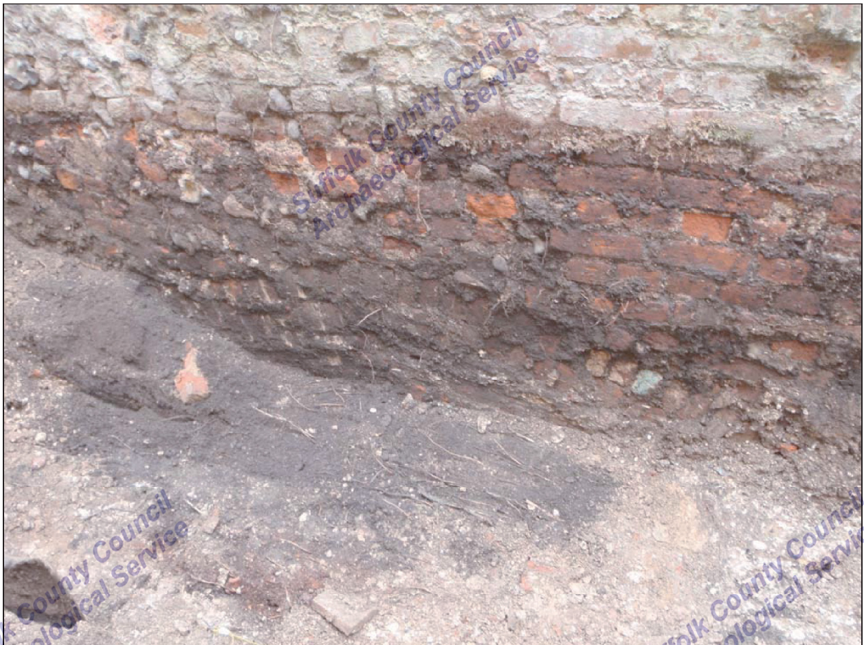
Plate 2. Arch built in yard wall to strengthen it where it crossed pit 0019
