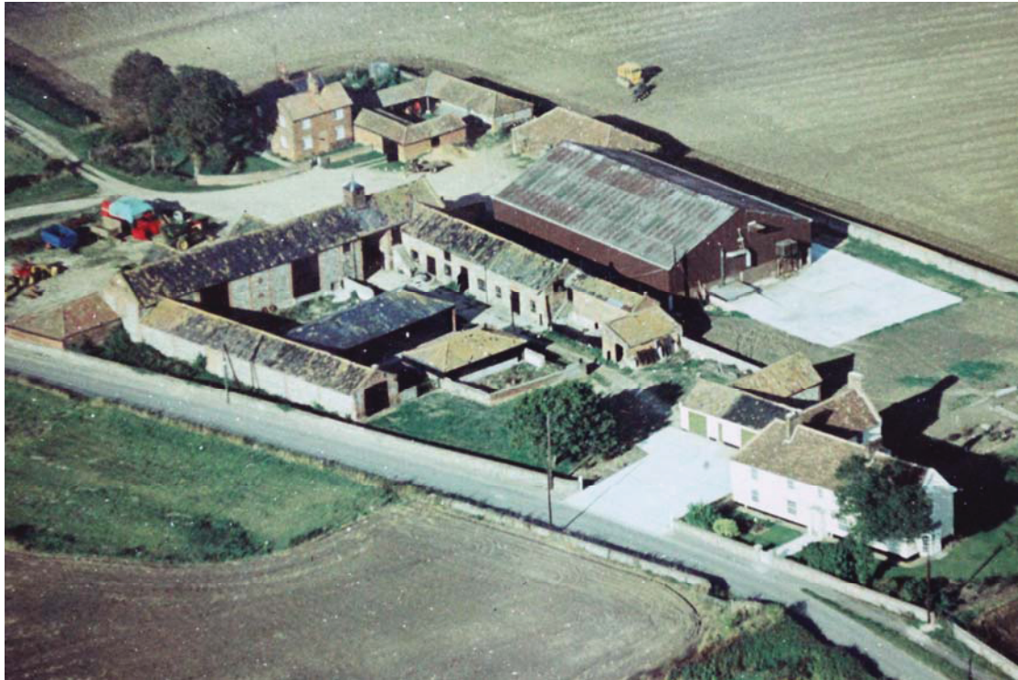
A2.1 Aerial view of site before conversion from south-west (dated 1972) showing farmhouse to right and single-storied linear shed to left (note black-painted vehicle doors in gable). Original in possession of owner.
