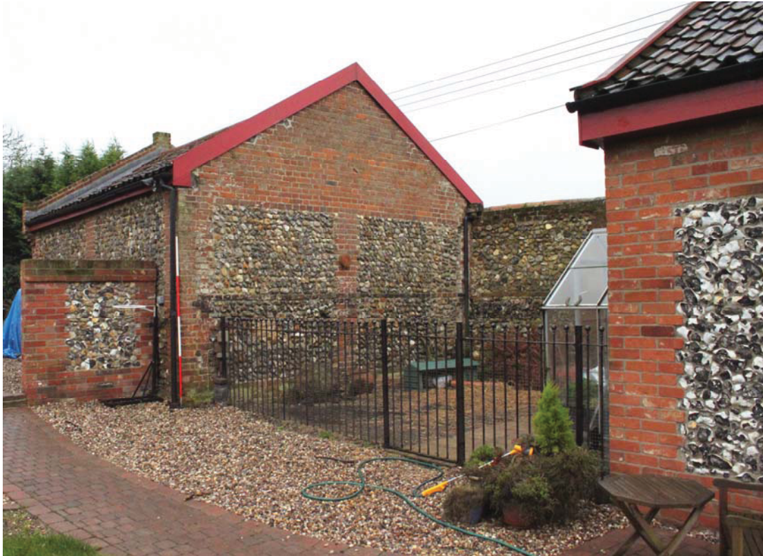
A2.5 Exterior of shed from north-east showing its truncated northern gable with the modern extension to its surviving northern section visible to right
