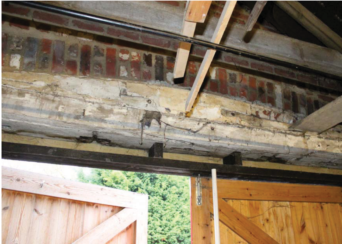
A2.9 Detail of re-used cambered medieval tie-beam above southern entrance doors showing empty pegged mortises in its underside
