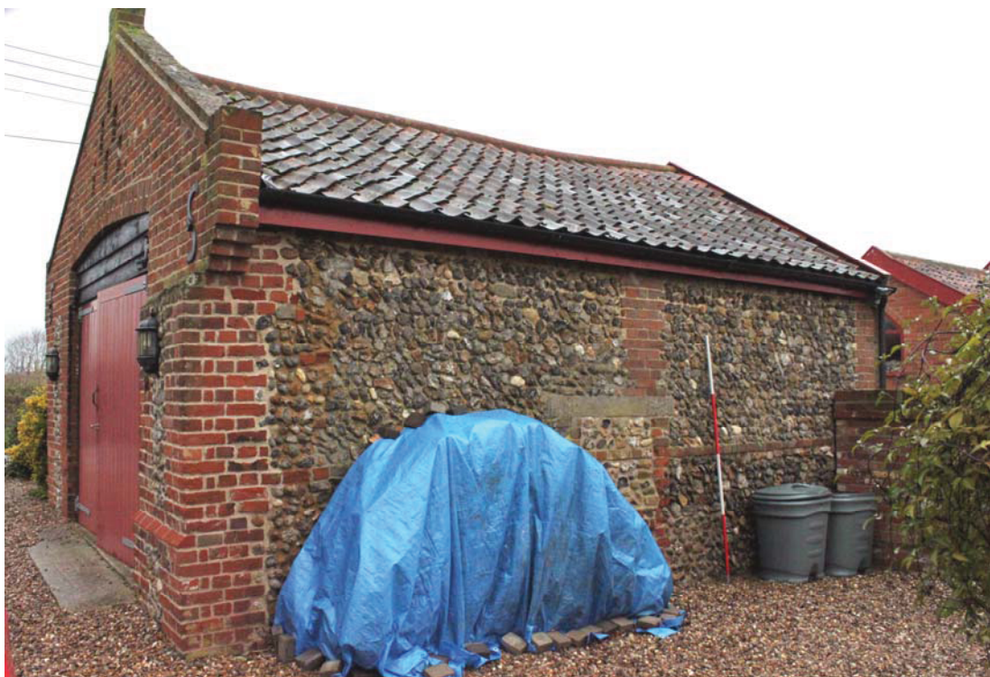
A2.4 Exterior of shed from south-east showing southern gable to left and blocked central aperture of eastern elevation to right. The shed formerly continued further to the north (right) but was partly demolished during the conversion of 2000 and the gable shown here to the extreme right is a more recent 'extension' to its extant northern end.
