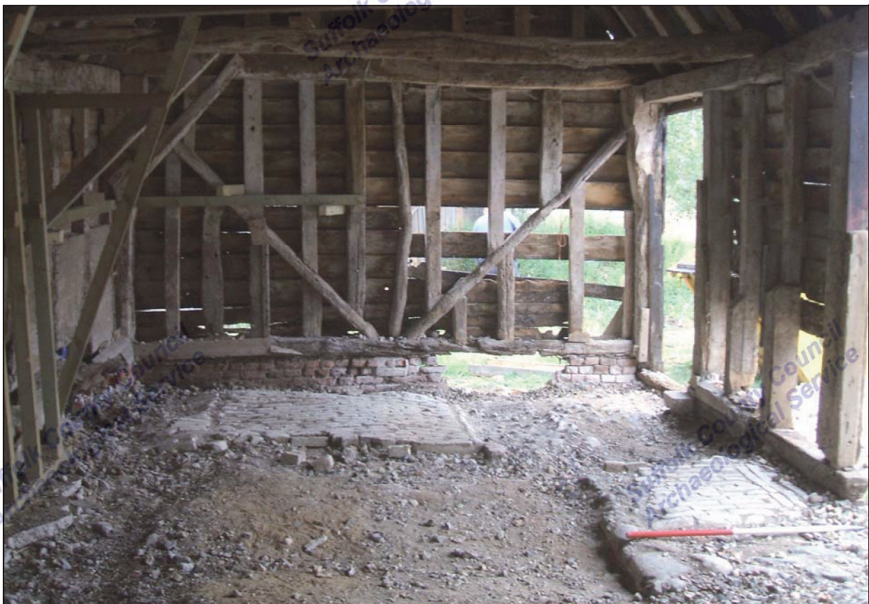
Figure 6. Interior of north barn, facing east, showing 0030 and 0031
