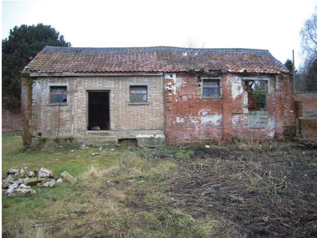
A2.3 Shed 1. External southern elevation showing 20th century brickwork to left and original brickwork with secondary windows to right
