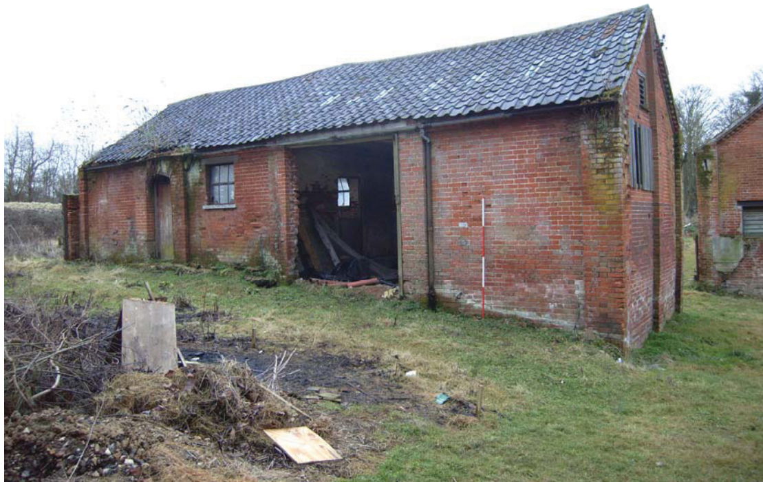
A2.4 Shed 1. External northern elevation showing secondary opening to right with original door to left
