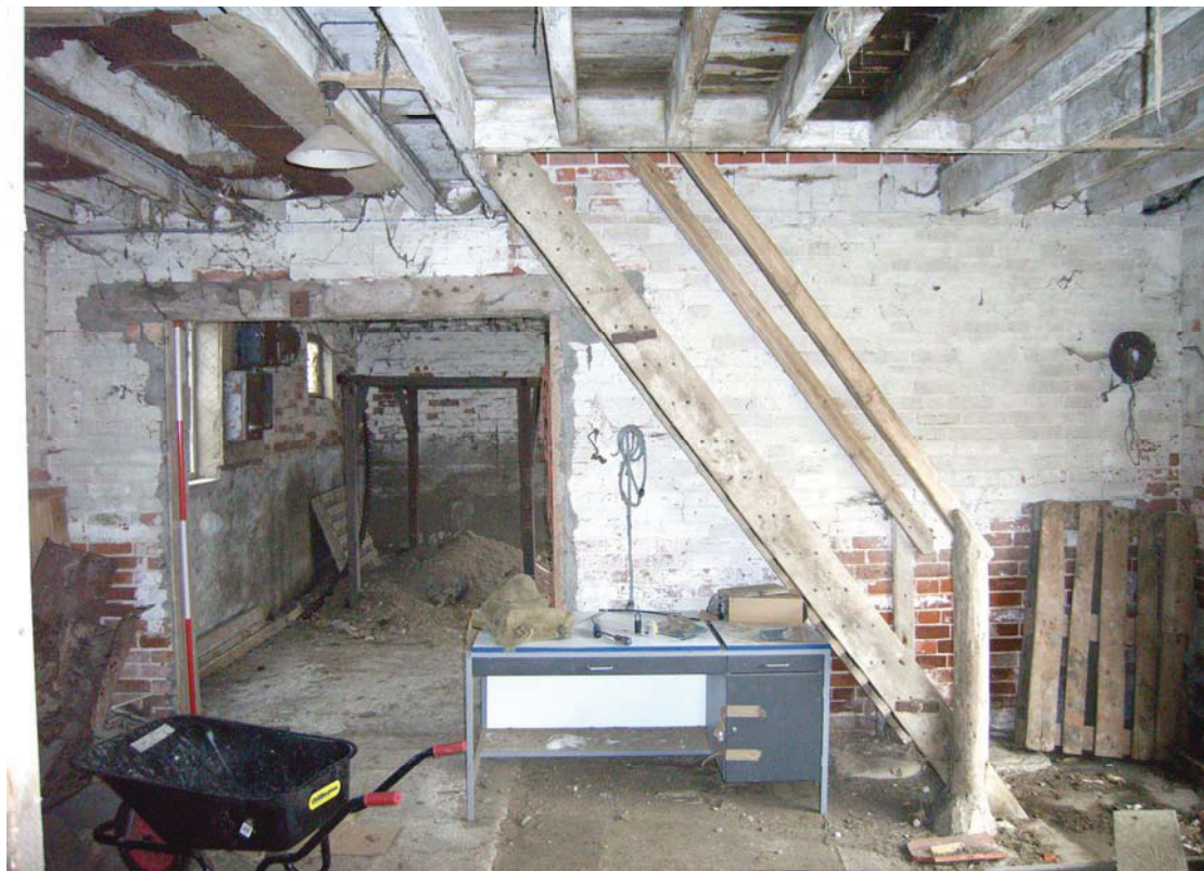
A2.8 Granary 2. Secondary stair in central compartment seen from south
