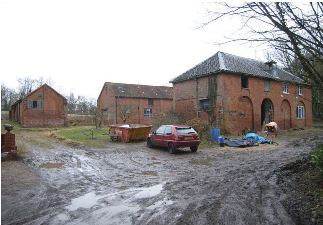
A2.2 General view of site from entrance to north-west showing Georgian stable to right with shed 1 to left and granary 2 in centre
