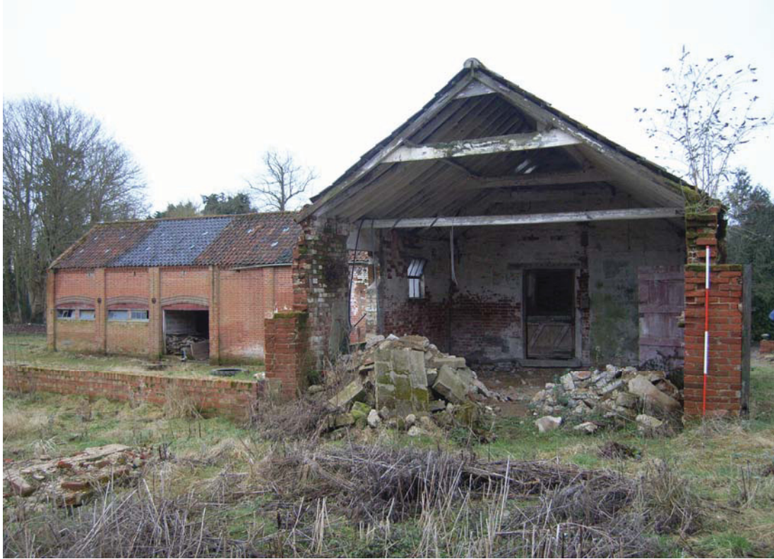
A2.5 Shed 1. Exterior of truncated eastern gable showing granary 2 to left
