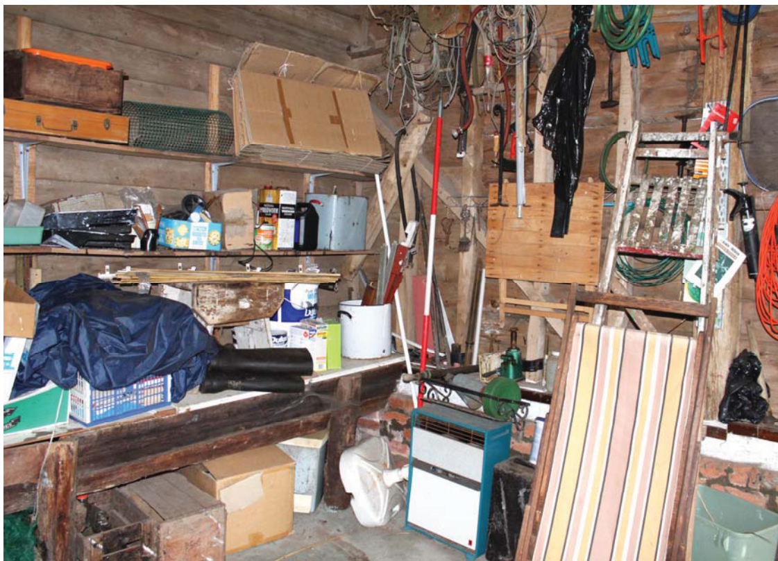
A2.10 North-eastern internal corner of cow shed (D) showing low boarded cattle manger beneath modern shelving against barn wall to left and the diagonal rail of a missing hay rack in centre (to left of half-metre scale rod).
