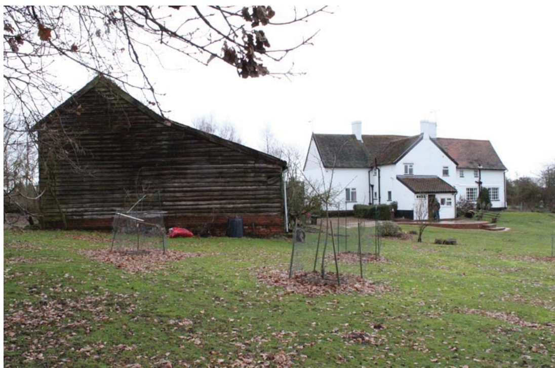
A2.1 General view of site from west showing barn with contemporary lean-to sheds to left and farmhouse to right. The late-16 th or early-17 th century farmhouse contains a parlour to the right with a central hall and a 20 th century extension beyond the small chimney to left. The central wing was added in the mid-19 th century.
