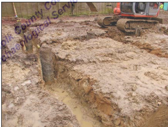
Plate III: Ground beam trenches excavated for plots 7 and 8
