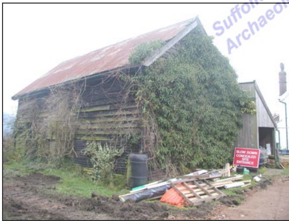
Plate I: Timber workshop on the site of plots 1, 2 and 3, prior to demolition
