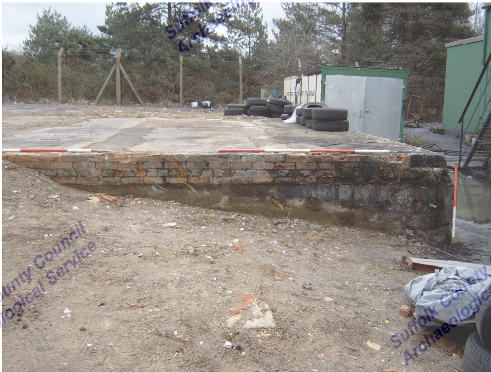
Figure 7 South-west corner of platform
