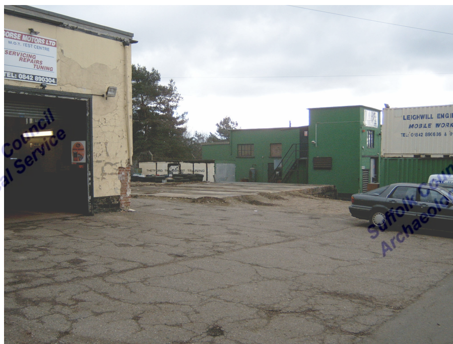
Figure 3 General view looking south-east
