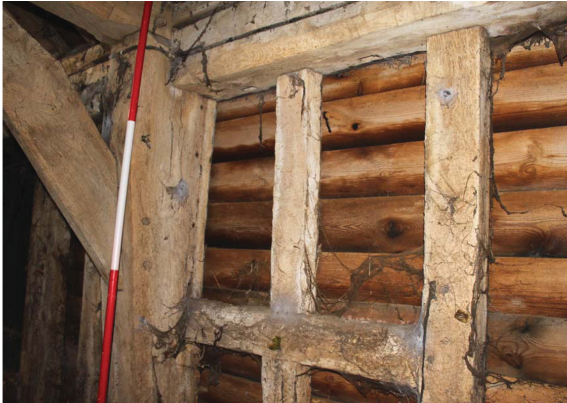
A2.11 Detail of Original loft window in northern internal elevation of bay C showing rectangular mullion mortises and original sill.
