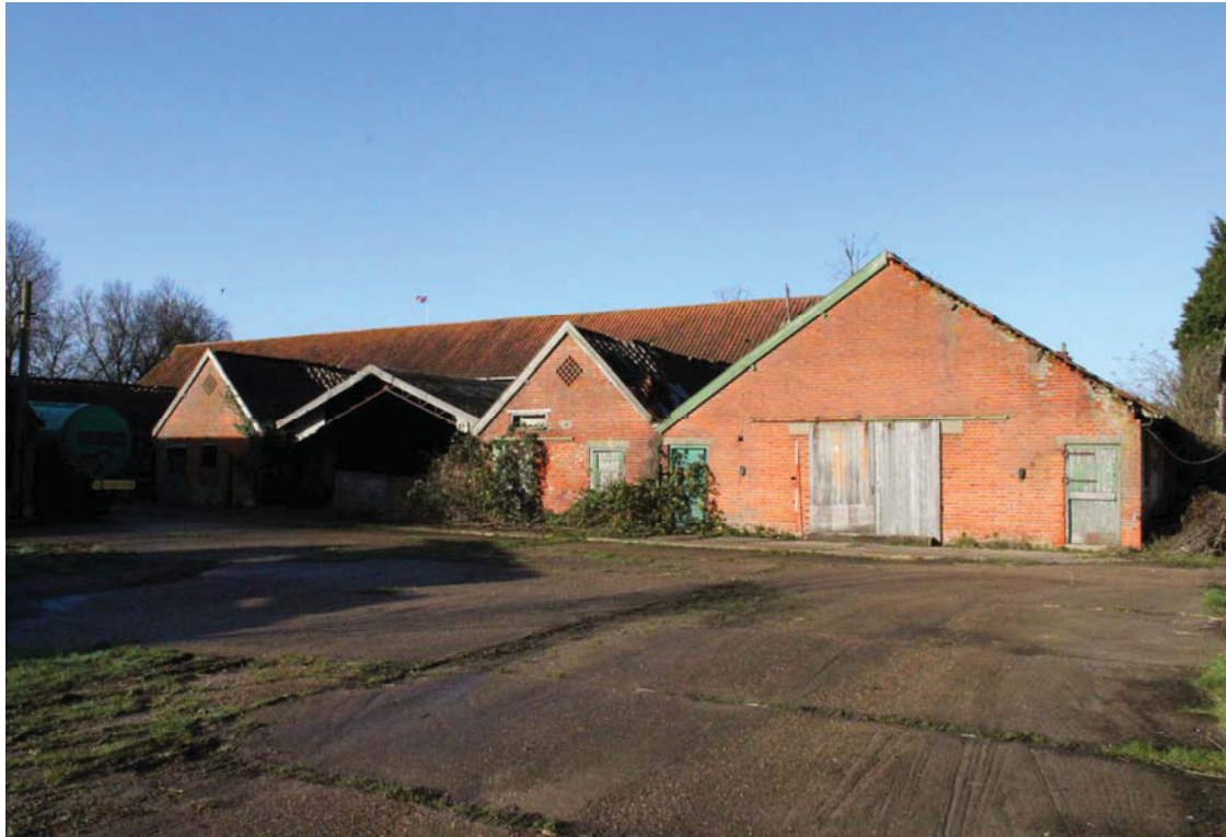
A2.3 Southern exterior of barn (1) showing two of the three mid-19 th century brick yard shelter-sheds to the left (3 & 4, each with an enclosed southern feed store with a lozenge-shaped ventilation aperture at its gable) and the early-20 th century cow shed or covered cattle yard (5) to right.
