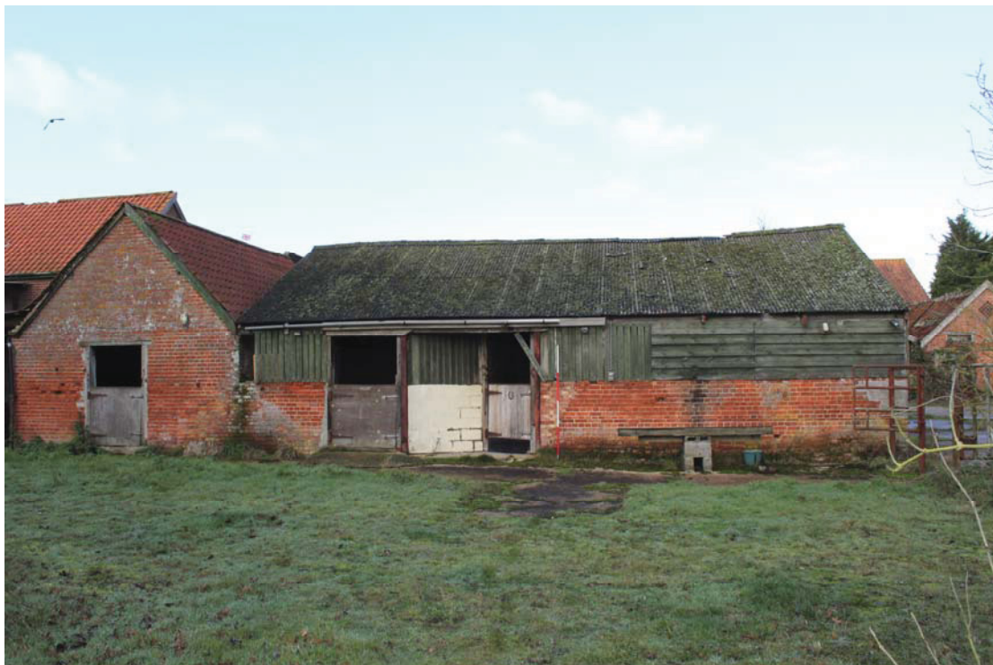
A2.14 Southern exterior of cow shed and covered yard (9) recently converted into block-work stable units, showing the cartlodge/granary (6) in rear to left and the eastern end of the barn to the right.
