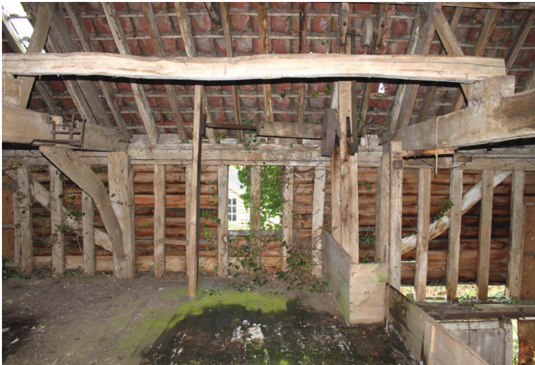
A2.10 Northern interior of bay F (above section 1b) showing the externally trenched braces which radiated from the original barn's rear door. Note the feed milling mechanism to the right (consisting of a drive shaft, wooden belt axle and iron wheel)
