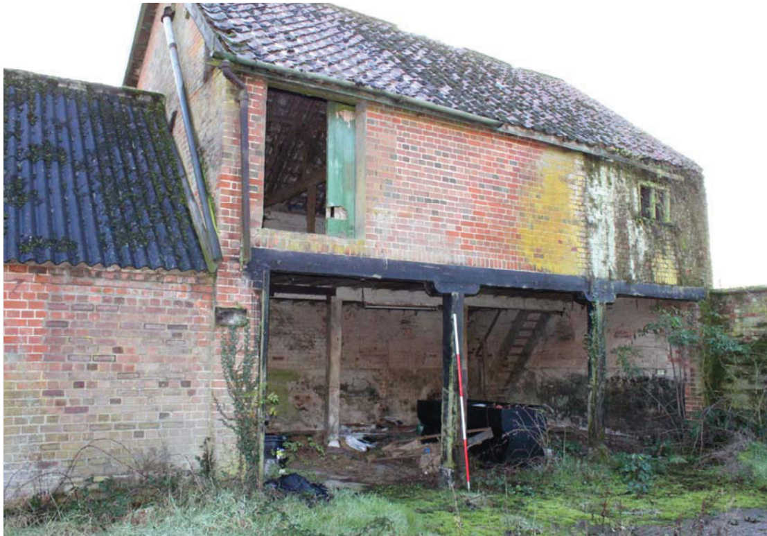
A2.13 Northern exterior of mid-19 th century cartlodge/granary (6) showing original open arcade and inserted loading door to first-floor (converted from a window). The original access from Wingfield Castle has been blocked by the 20 th century wall shown to the right, and the shelter shed now converted into a milking parlour (7) is visible to the left.
