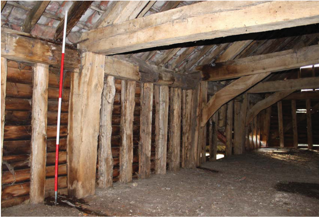
A2.9 Detail of from north-east of the open truss between bays C and D which consists of a storey post and tie-beam (both without chamfers) but lacks arch-braces. The tie-beam contains 10 stud mortises in its upper surface but none beneath. A brick partition at this point would have divided the original stable and loft from the open barn.
