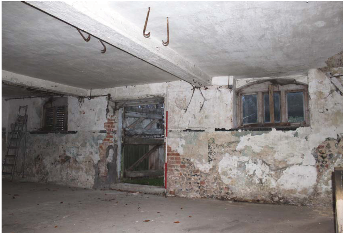
A2.6 Southern interior of stable (1) showing central yard door flanked by windows and showing diagonal strut of former hay rack against western elevation to right.
