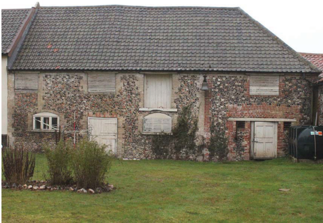
A2.3 Southern exterior of flint stable (1 to left) and later coach house subsequently converted into a game store (2 to right). Note blocked arched doorway of coach house and original first-floor loading door of stable to extreme left.
