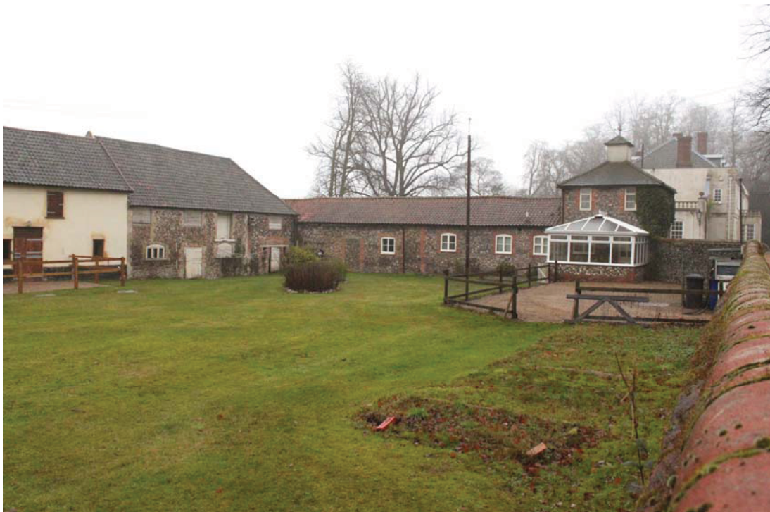
A2.2 General view of former stable yard from west showing from left to right: clay-lump mid-19 th century stable, early-19 th century flint rubble stable with later coach house to right (1 & 2), single-storied modern coach house (6), converted single-storied shed and probable granary (with turret clock), Rushford Hall (in rear) and yard wall to north of drive.
