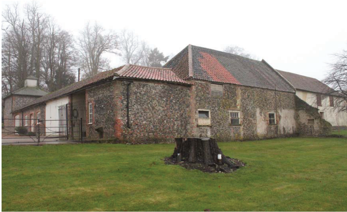
A2.5 General view of former stable yard from west showing from left to right: converted single-storied shed and probable granary (with turret clock), single-storied modern coach house (6), single-storied tack room now converted into kennel (at corner), early-19 th century flint rubble stable with later coach house to left (1 & 2) – showing remains of lean-to rack room to right – and clay-lump mid-19 th century stable to extreme right.
