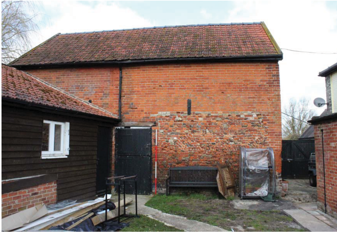
A2.5 Southern exterior of stable showing original central entrance with recently converted northern shed (2) to left and western gable of Public House (5) to right.
