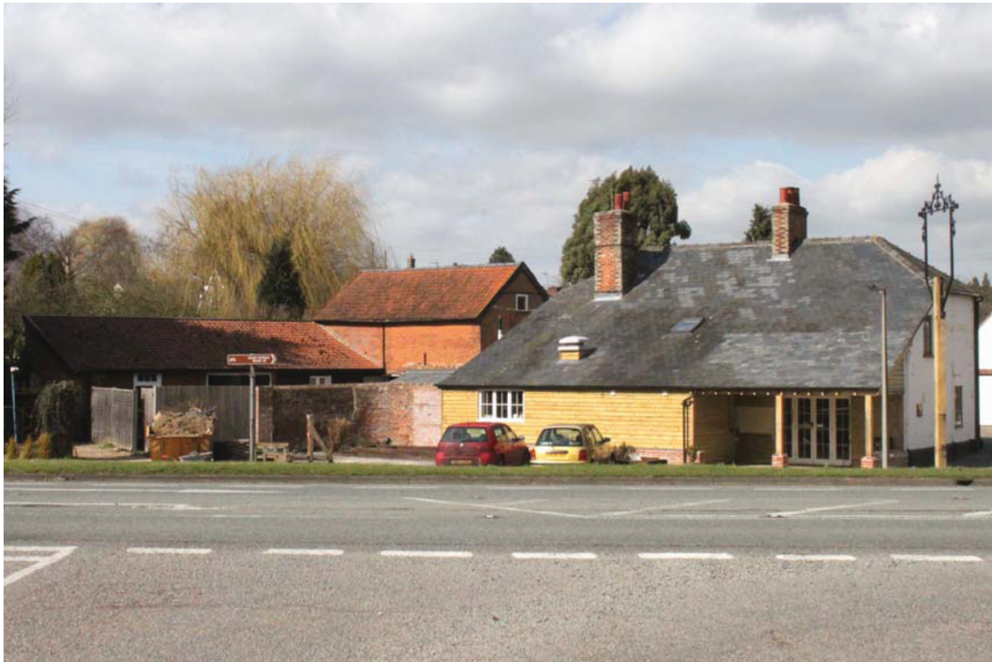
A2.1 General view from modern A134 to south-east showing red-brick stable (1) and single-storied range of sheds (2-4) to left & rear elevation of Rose & Crown Public House (5) to right
