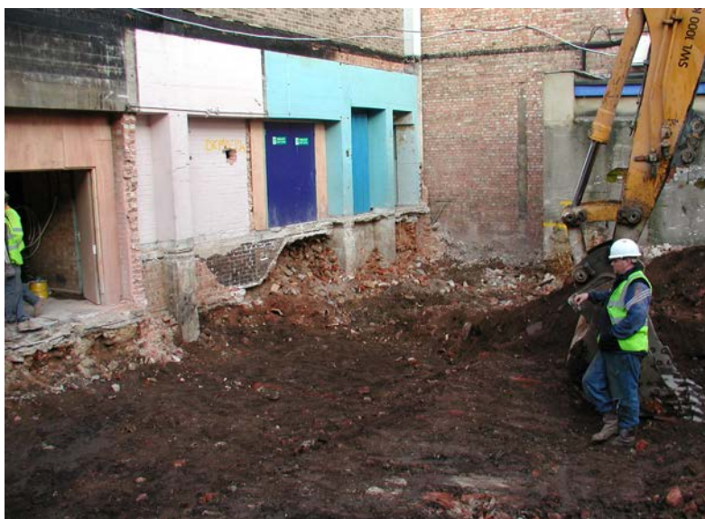
Plate 1: View of stripped site, looking north east.
