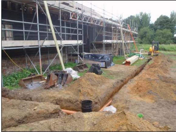
Plate 9. Drain run to NW
