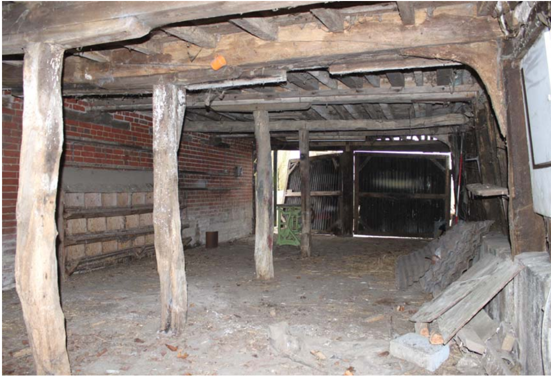
Illus. 7. Interior of lower storey from north showing axial Sampson posts and brick eastern elevation to left. The original ceiling joists of the northern bay shown here are tenoned to the binding joists.
