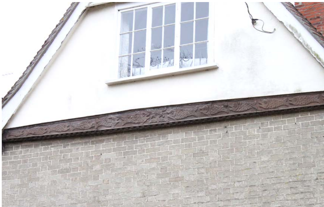
Illus. 2. Detail of the highly unusual and ostensibly authentic early-17 th century northern tie-beam of Ringshall House, carved with fish. A similar tie-beam with drop finial survives to the south. Included for site context.
