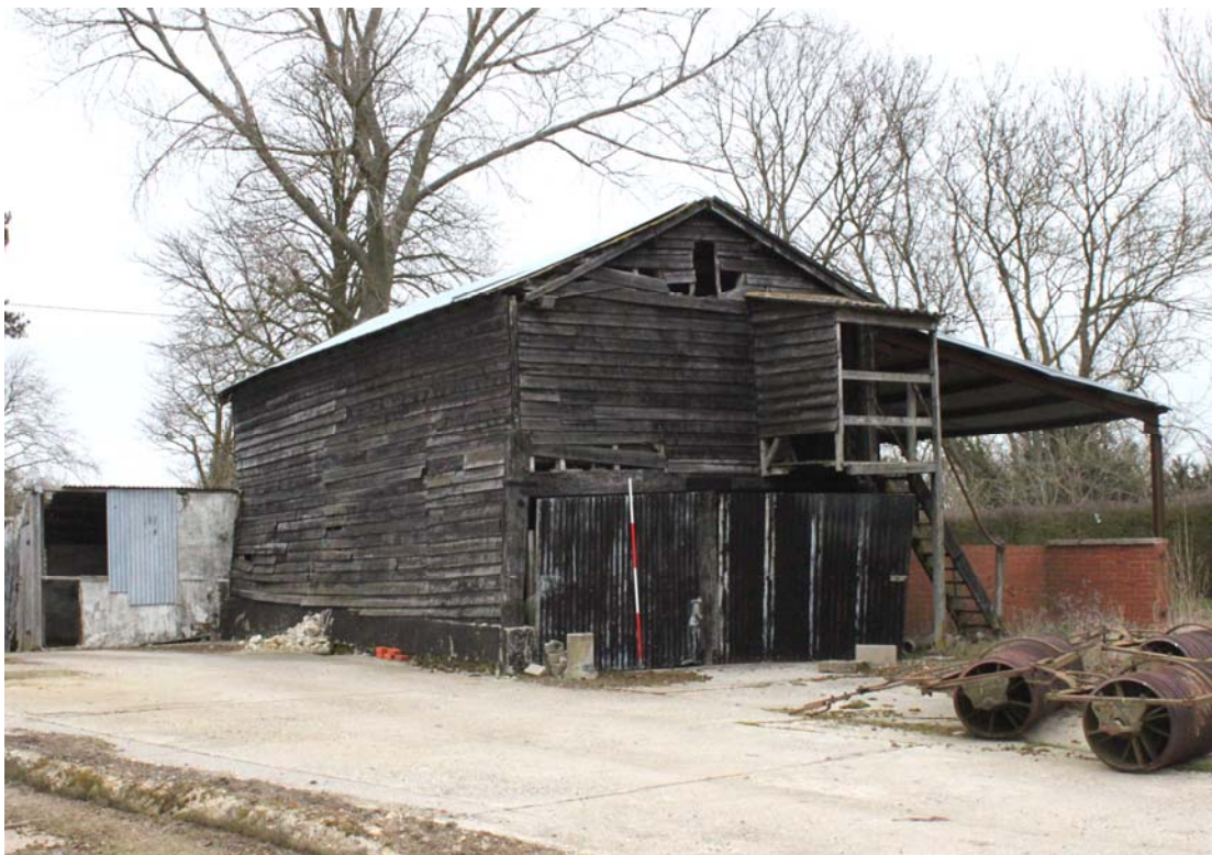
Illus. 4. Exterior of granary from south-west showing rebuilt external stair against southern gable and roadside vehicle shelter to right. Note corrugated iron vehicle doors to ground floor of gable.
