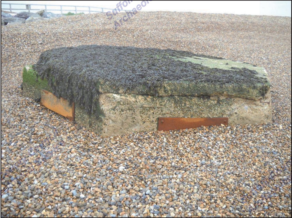
Plate 12. BAW 153 after completion of new sea defences, facing west (Courtesy of the Environment Agency)
