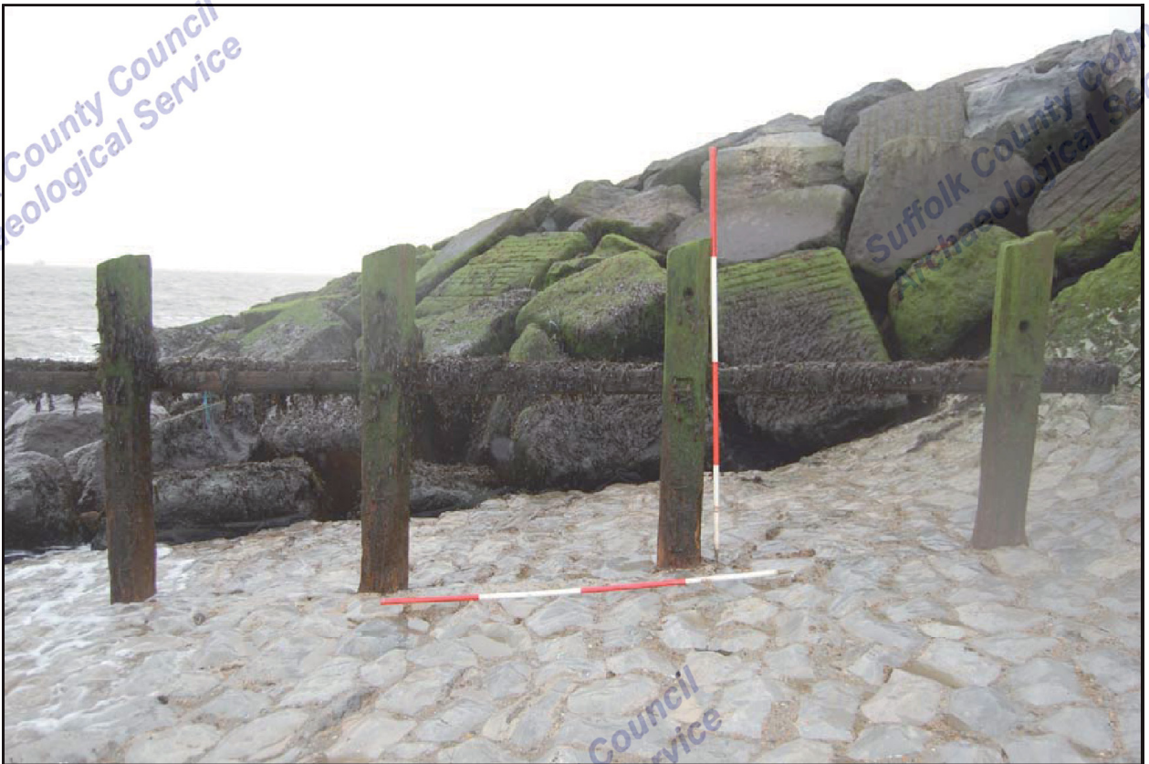
Plate 5. BAW 164, Groyne 1, facing south
