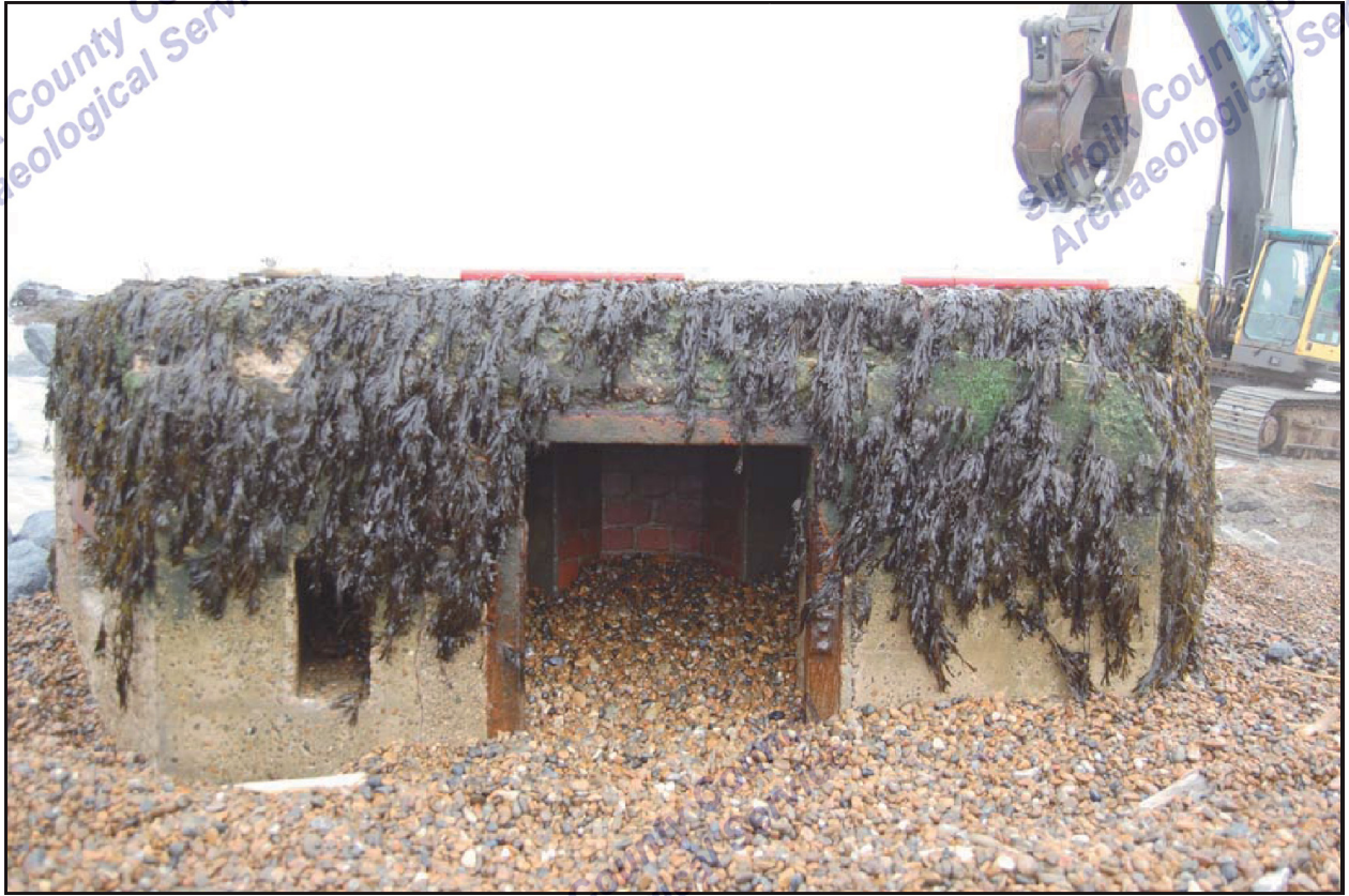
Plate 1. BAW 153, doorway elevation of pillbox, facing south-east
