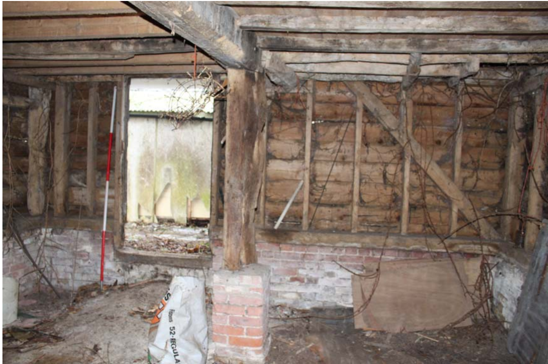
Illus. 7. Eastern internal gable showing 20 th century framing with a door opening towards the farmhouse. The central post is an insertion of the 19 th century which supports the end of the 17 th century axial ceiling joist where it would formerly have abutted a chimney.
