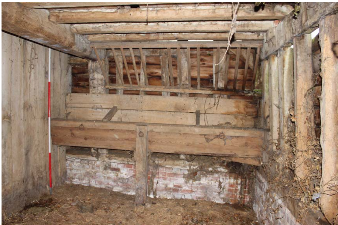
Illus. 10. The feeding trough and hay rack at the western end of the southern internal elevation (at horse height), showing the western gable to the right. Note the original diamond mullion window behind the rack, and evidence for additional mullions in the gable. The boarding to the left is a stall divider.
