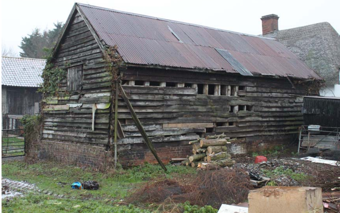
Illus. 3. Exterior of stable (1) from south-west showing loft loading hatch in western gable to left and farmhouse to right.
