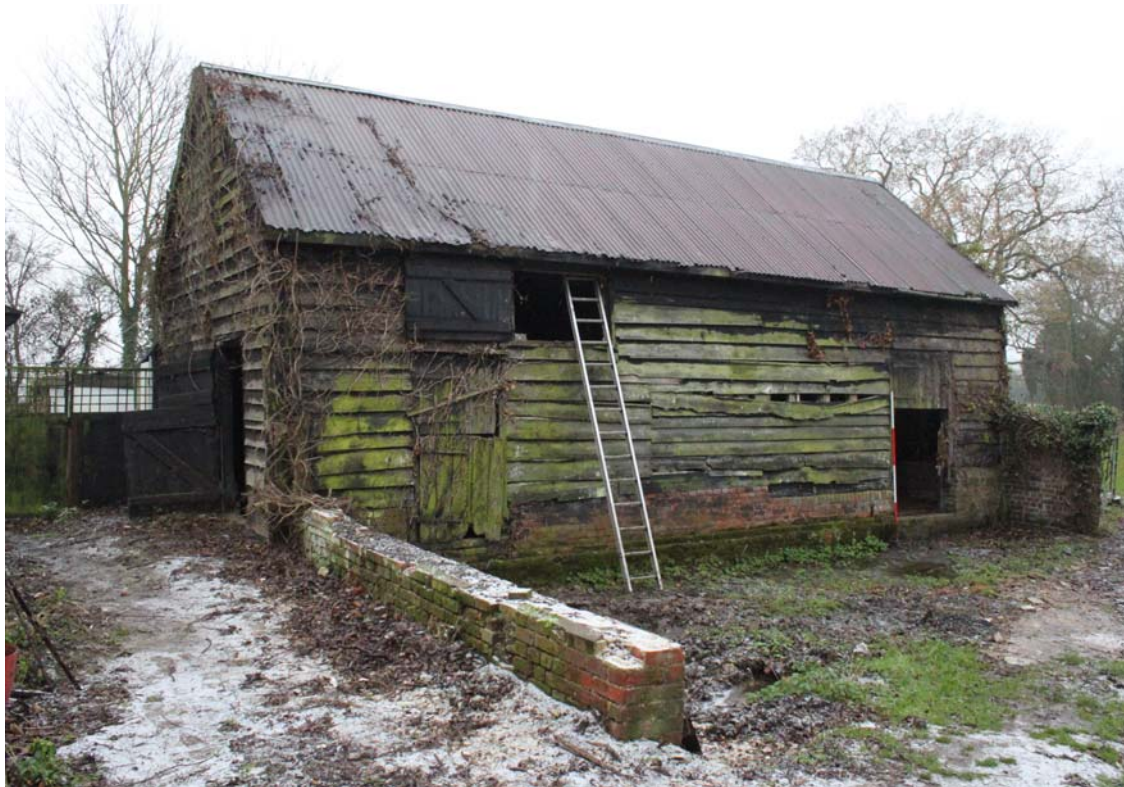
Illus. 4. Exterior of stable from north-east showing half-hung entrance doors to yard, loading door to eastern loft and door in eastern gable to left.
