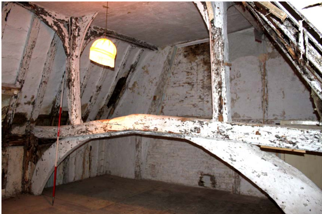
Illus. 2. The queen-post open-truss of the 15 th century open hall in the farmhouse (2) seen from the low-end to the north-west. The whitewash conceals heavy sooting. Included for site context.
