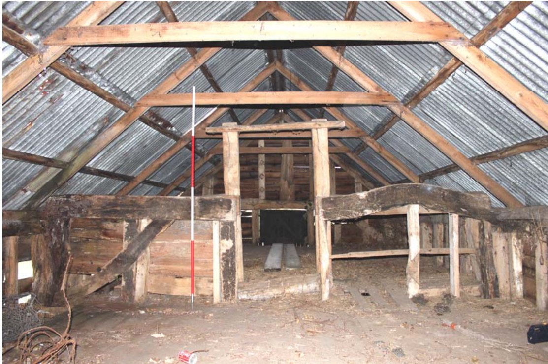
Illus. 5. Interior of eastern loft from east showing the upper part of the sooted medieval 'high-end' partition which divides the building into two halves. Note the original wall brace to the left and the bow in the tie-beam to right. This bow would have reflected an original doorway beneath, which explains the absence of a right-hand wall brace. The central door is an insertion of the 17 th century and the roof is modern.
