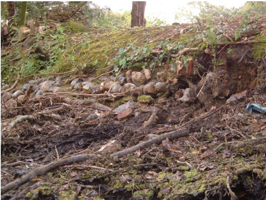
Plate 5. Detail of revetment wall
