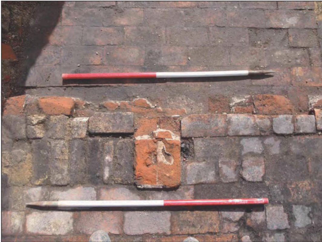
Plate XI. View of dividing Wall 0025 and buttress on its northern side
