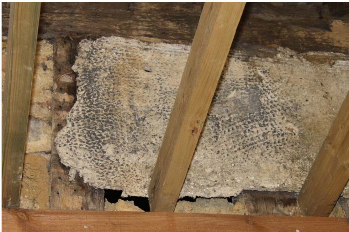
Illus. 12. Textured pargeing to western exterior of barn's northern bay, seen through the modern ceiling joists of the lean-to shed (5) and showing the roof-plate above. This decorative plasterwork probably dates from the 18 th century and lies above a lower tier of weatherboarding. The weathering to the studs suggests they were originally exposed externally.
