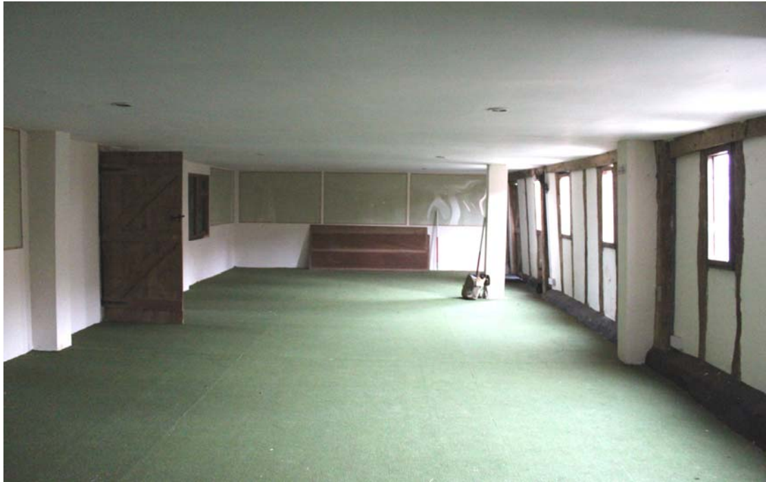
Illus. 5. Interior from north of central section of barn (1) showing modern ceiling and windows with original framing in western elevation to right. The partition to the left is a modern insertion forming an internal corridor against the barn's eastern elevation.
