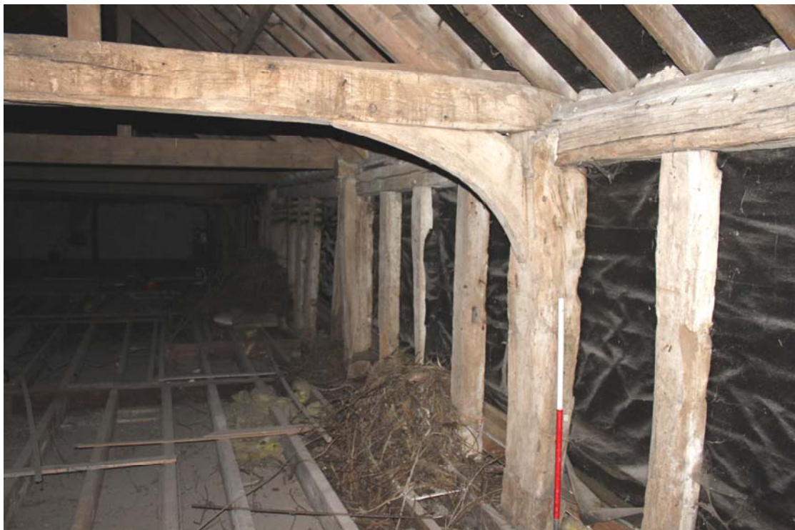
Illus. 10. The original tie-beam and brace between the two bays of the former hay loft, as seen from the south (i.e. above the ground-floor WCs). The opposite (western) brace has been removed.
