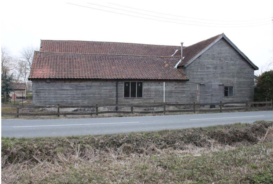
Illus. 2. Eastern external elevation showing gabled porch (2) to right and lean-to shed (3) left. The right-hand half of the lean-to shed was originally an open-sided cart lodge. The roof of the main barn (1) is visible in the rear.
