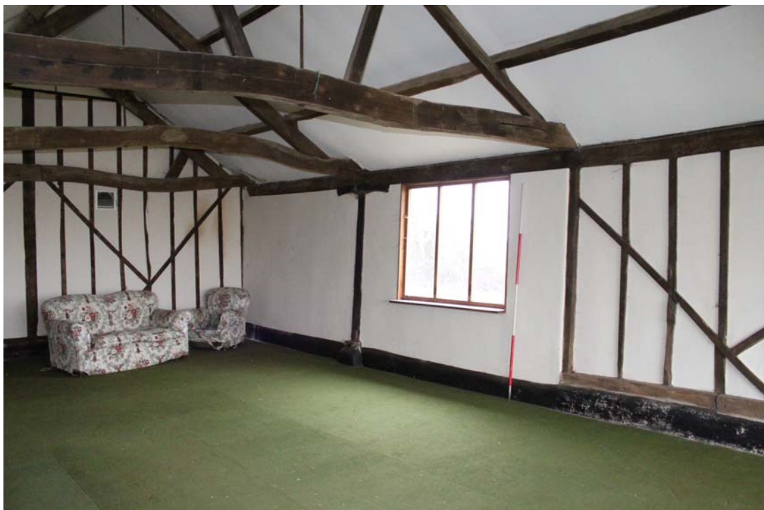
Illus. 4. Interior of eastern shed (3) from south-west showing the arcade-post of the originally open-sided northern half of the eastern internal elevation in the centre. The missing partition beneath the tie-beam which divided this roadside cart shed from the enclosed shed in the foreground is still shown on the modern Ordnance Survey (figure 1).
