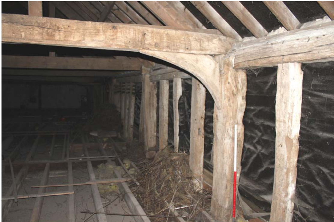
Illus. 10. The original tie-beam and brace between the two bays of the former hay loft, as seen from the south (i.e. above the ground-floor WCs). The opposite (western) brace has been removed.
