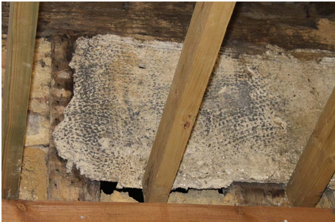
Illus. 12. Textured pargeing to western exterior of barn's northern bay, seen through the modern ceiling joists of the lean-to shed (5) and showing the roof-plate above. This decorative plasterwork probably dates from the 18 th century and lies above a lower tier of weatherboarding. The weathering to the studs suggests they were originally exposed externally.
