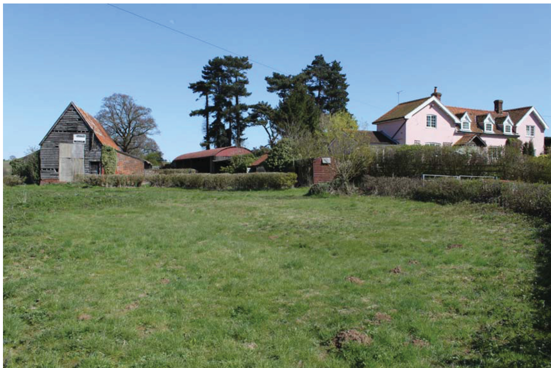
Illus. 2. General view of site from west showing farmhouse (11) to right and barn (1) to left. The house was ostensibly rebuilt in circa 1920 but occupies the site of a predecessor shown on 19 th century maps and may contain earlier fabric.
