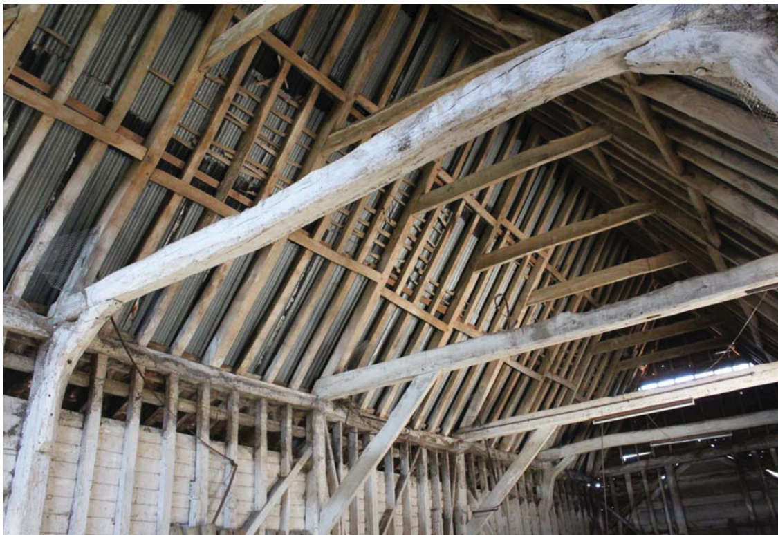
Illus. 8. The intact and impressive staggered butt-purlin roof structure of the barn (1) seen from the south-west and showing the central arch-braces between the original knee-braces of the outer bays. Note the surviving thatch battens beneath the 20 th century corrugated iron.
