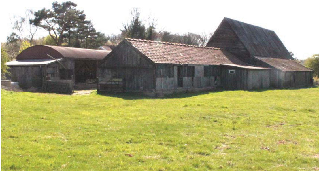
Illus. 1. General view of site from north-east showing the early-19 th century barn (1) to right with late-19 th century lean-to sheds (2 & 6) and early-20 th century pantiled milking parlour (5) in centre. The cattle shed (9) is visible in the rear.
