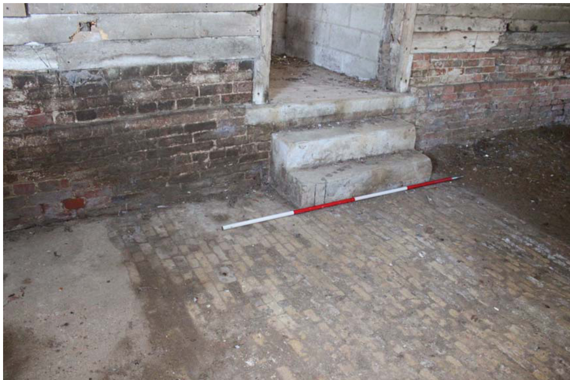
Illus. 10. Detail from north of the brick threshing floor in the lean-to shed (2) with the secondary door in the barn's central bay to the rear.
