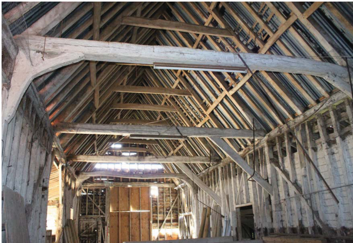
Illus. 6. Original roof structure of barn (1) seen from the east and showing the arch-braces to the tie-beams flanking the central threshing bay combined with bolted knee-braces to the outer trusses. The arch-braces to the south (left) have been removed.
