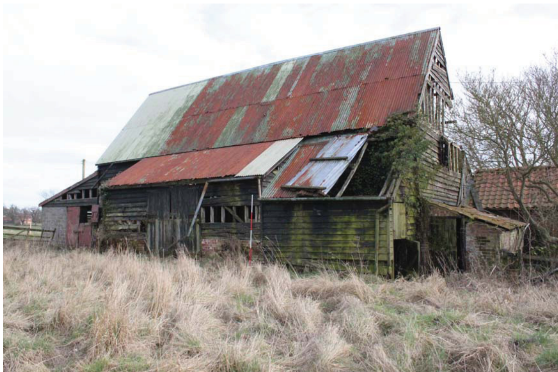
Illus. 4. Exterior of barn from north-west showing the original central lean-to porch (1a) with secondary lean-to shed (12) to right. A similar shed to the left of the porch has been demolished. The lean-to pig sty (2) against the barn's western gable is visible to the right and the lean-to bullock shed (3) against the eastern gable to the left. The brick feed store is shown in the rear to the right.
