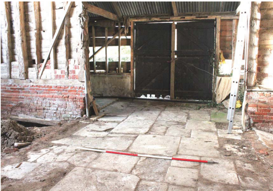
Illus. 8. Detail from south of the stone flag floor of the central bay of the barn (1) extending into the lean-to northern porch (1a).
