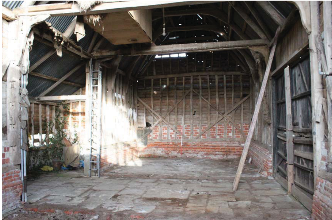
Illus. 5. Interior of barn (1) from east showing central southern entrance to left and lean-to porch (1a) to right. The central bay is flanked by tie-beams with original bolted knee-braces. Note the floor of stone flags in the same bay (possibly a later hard-standing rather than a threshing floor) and the diagonal primary braces of the eastern gable in the rear.
