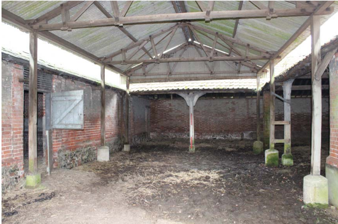
Illus. 5. Interior of covered yard (5) from south showing open arcade of shelter shed (3) in centre and to right, with curved corner of feed store (4) to extreme right and side door to barn (1) to left. The 'daisy wheel' apotropaic symbols lie to the extreme left.
