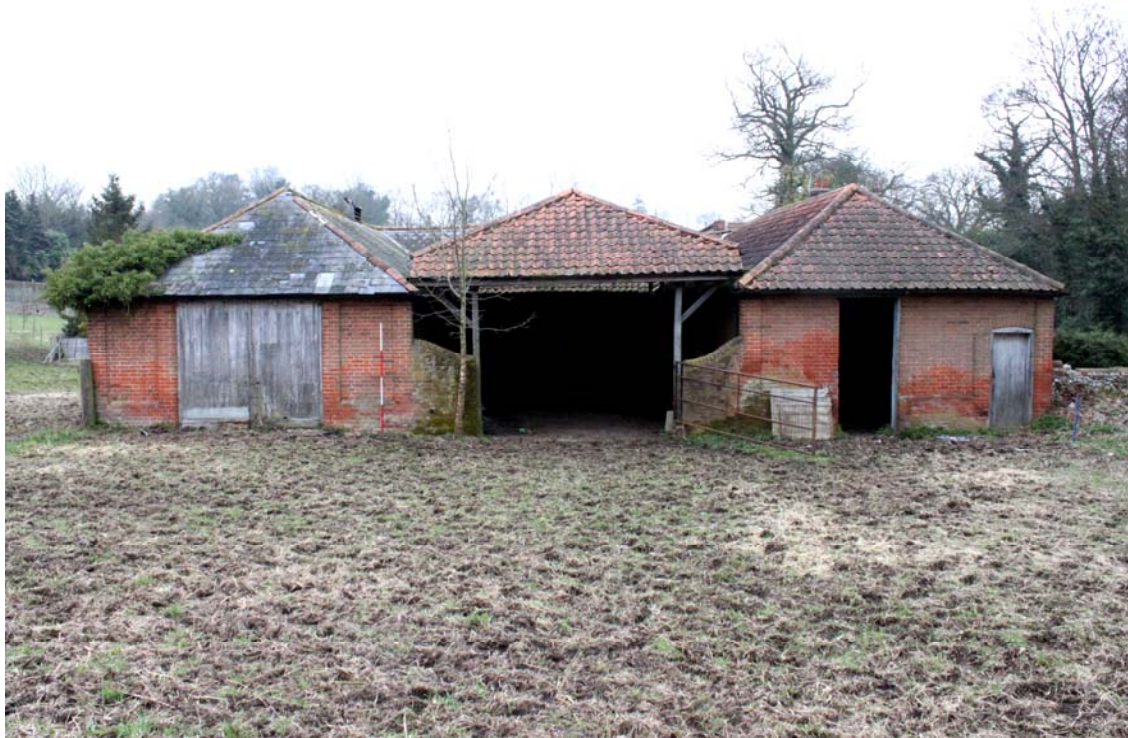
Illus. 4. Southern facade of barn complex showing 20th century of formerly open cattle yard (5) in centre, milling barn (1) with original double-doors to left and feed store (4) to right. The larger of the two doors to the feed store is secondary.
