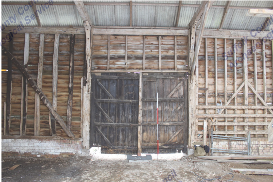
Illus. 9. Western interior of entrance bay C showing the reduced height of the entrance doors with original framing in bay D to left (with unusual re-used burnt timber) and rebuilt framing of the late-19 th or early-20 th century in bay B to right.
