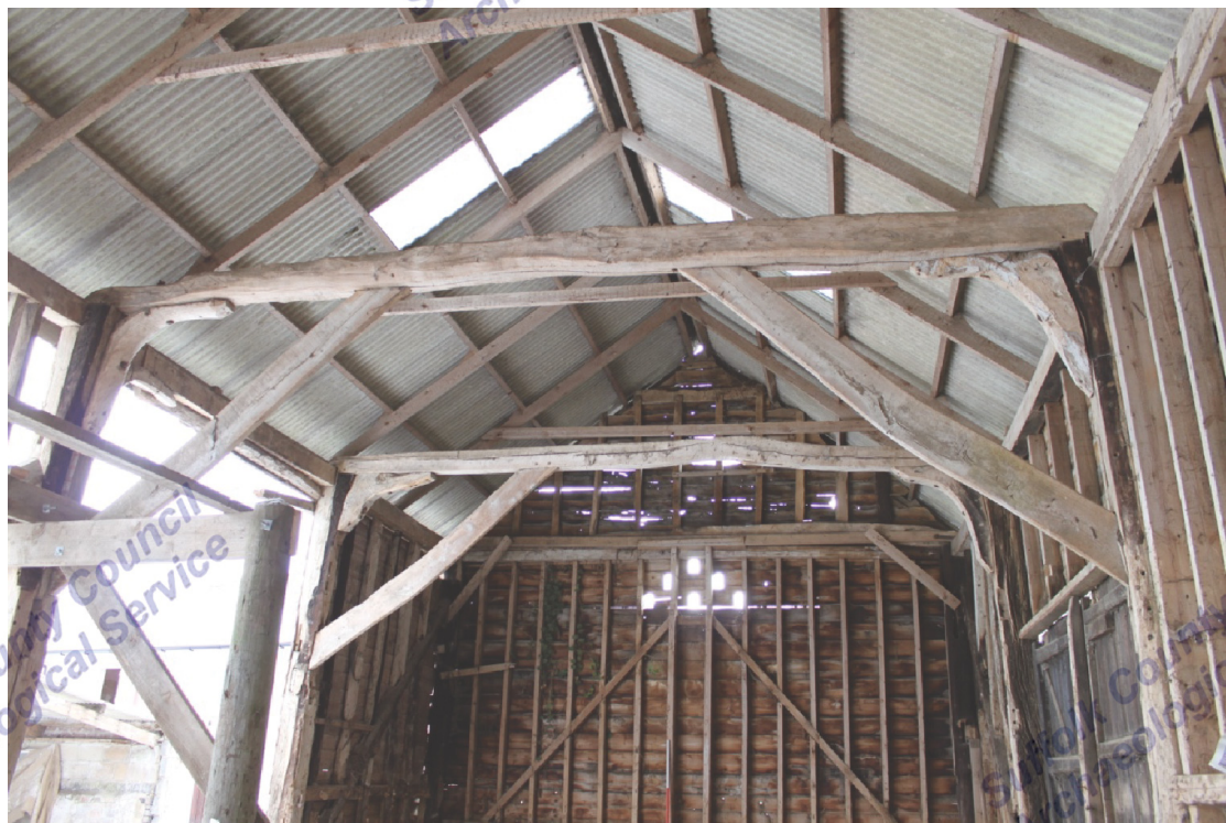
Illus. 8. Bolted knee-braces and reverse-cranked arch-braces of entrance bay C seen from north with 20 th century roof and rebuilt southern gable in rear
