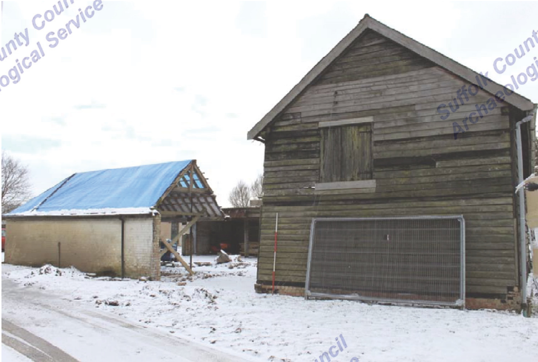
Illus. 5. Northern external gable of barn showing left loading door with brick shed (3) to left.
