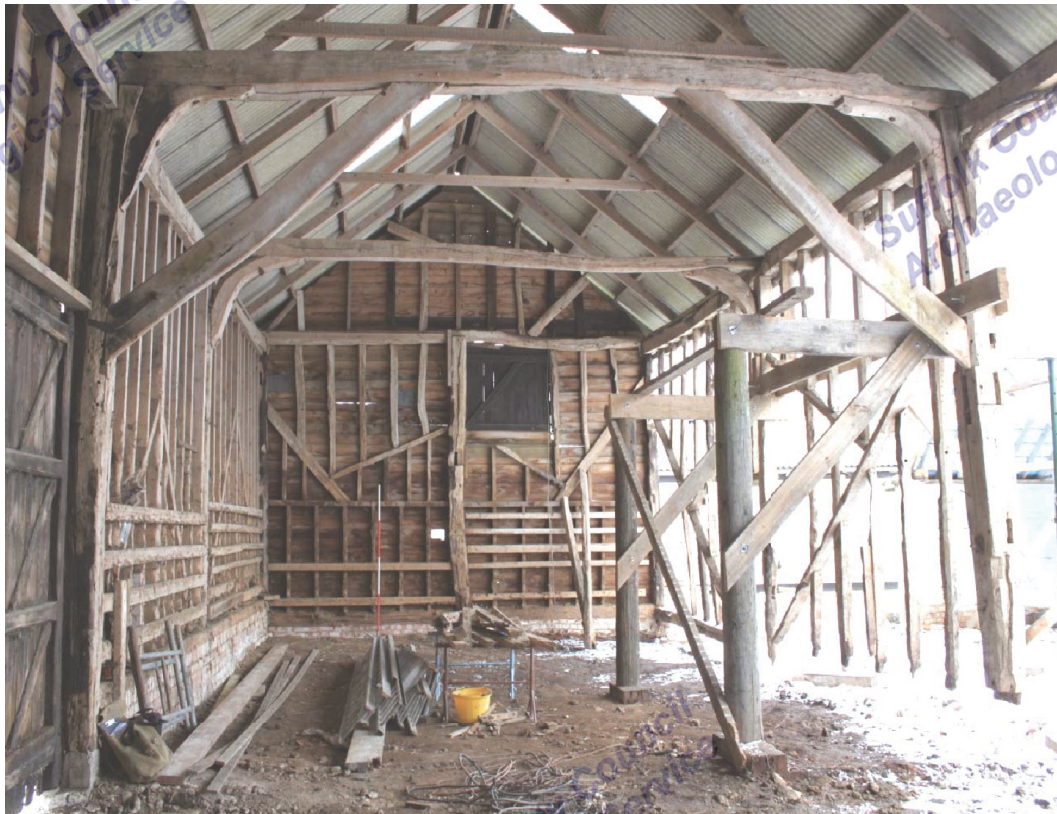
Illus. 7. General view of barn interior from south showing entrance bay C in foreground and the unusual combination of tenoned arch-braces and bolted knee-braces to its open trusses.
