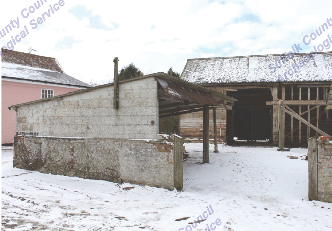
Illus. 3. Eastern yard entrance showing farmhouse & 20 th century block-work shelter shed (4) to left with eastern exterior of barn in rear.
