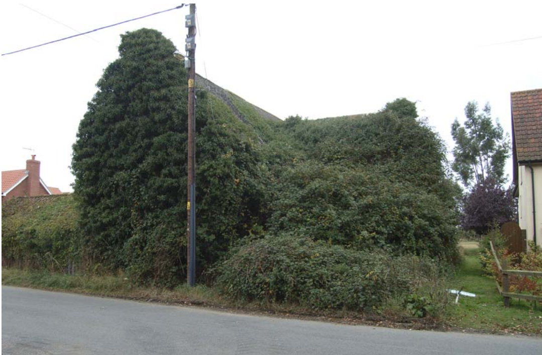
Illus. 2. Exterior from Mill Street to north showing the overgrown porch and lean-to shed (1a and 2) to the right. 'Hector's House' is shown in close proximity to the extreme right.
