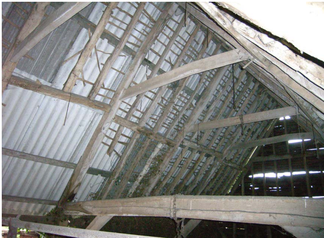
Illus. 8. Original roof structure of staggered butt-purlins seen from north-west, showing thatch battens and gap above eastern entrance to left which may relate to the additional porch shown on the title map.
