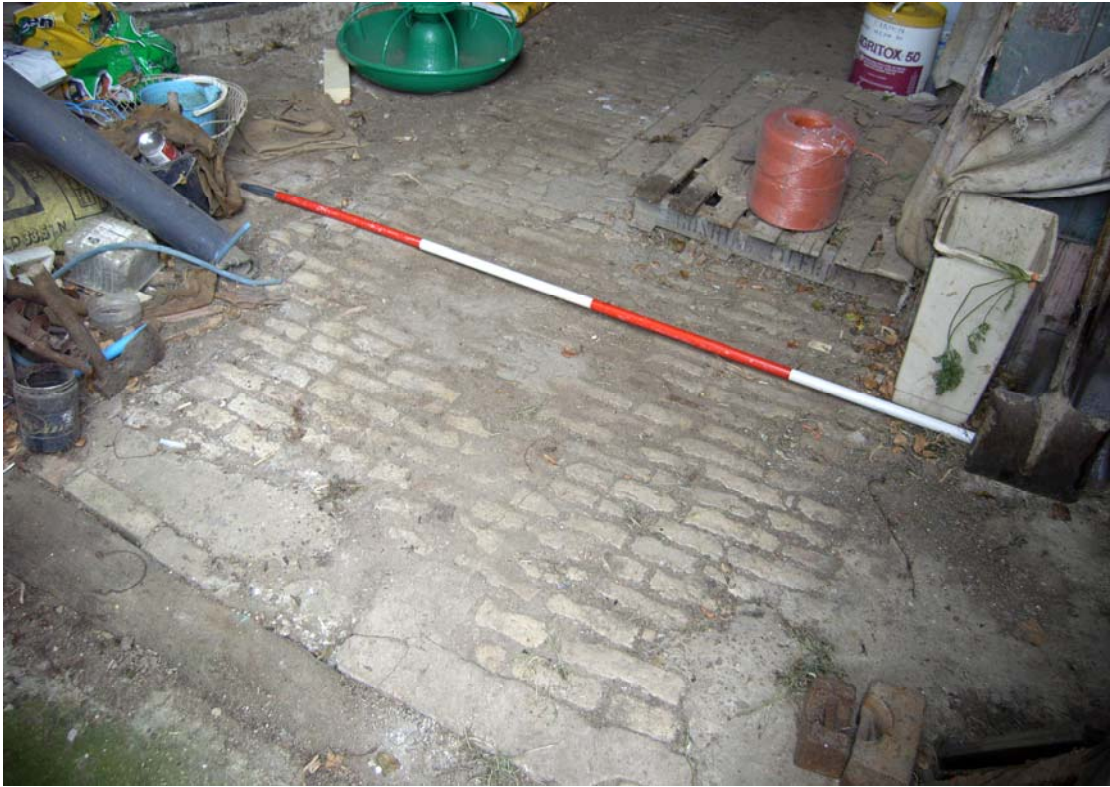
Illus. 5. Detail of gault brick threshing floor in central bay of barn seen from eastern entrance.
