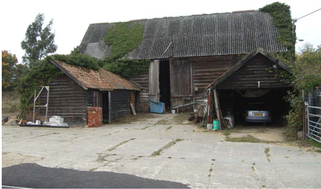
Illus. 3. Exterior of barn from east showing late-19 th century single-storied sheds 3 and 4 to left and right respectively.
