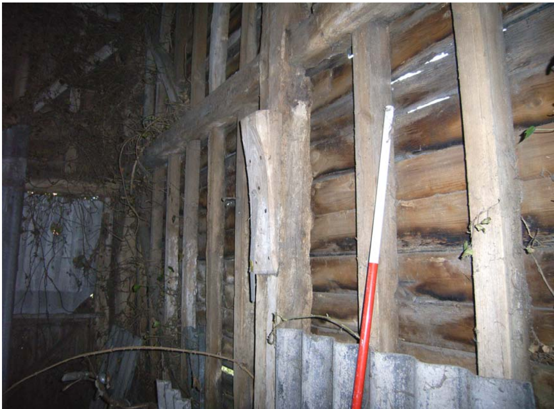
Illus. 10. Detail from west of nailed bracket on central post of southern gable for axial joist of removed stable ceiling, showing secondary stable door in eastern elevation to left.
