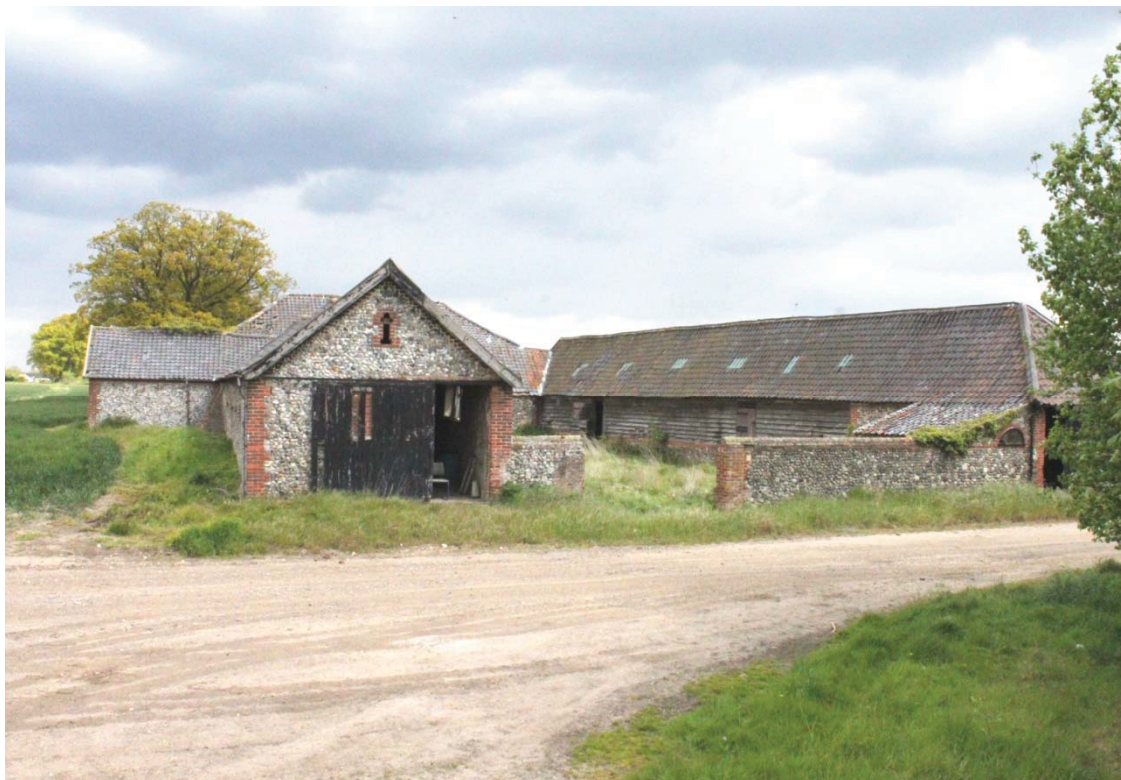
Illus. 2. Exterior of Barn 1 from south showing hipped roof of main barn (1) in rear with gable of stable (7) to left and cow shed range (3-5) to right.
