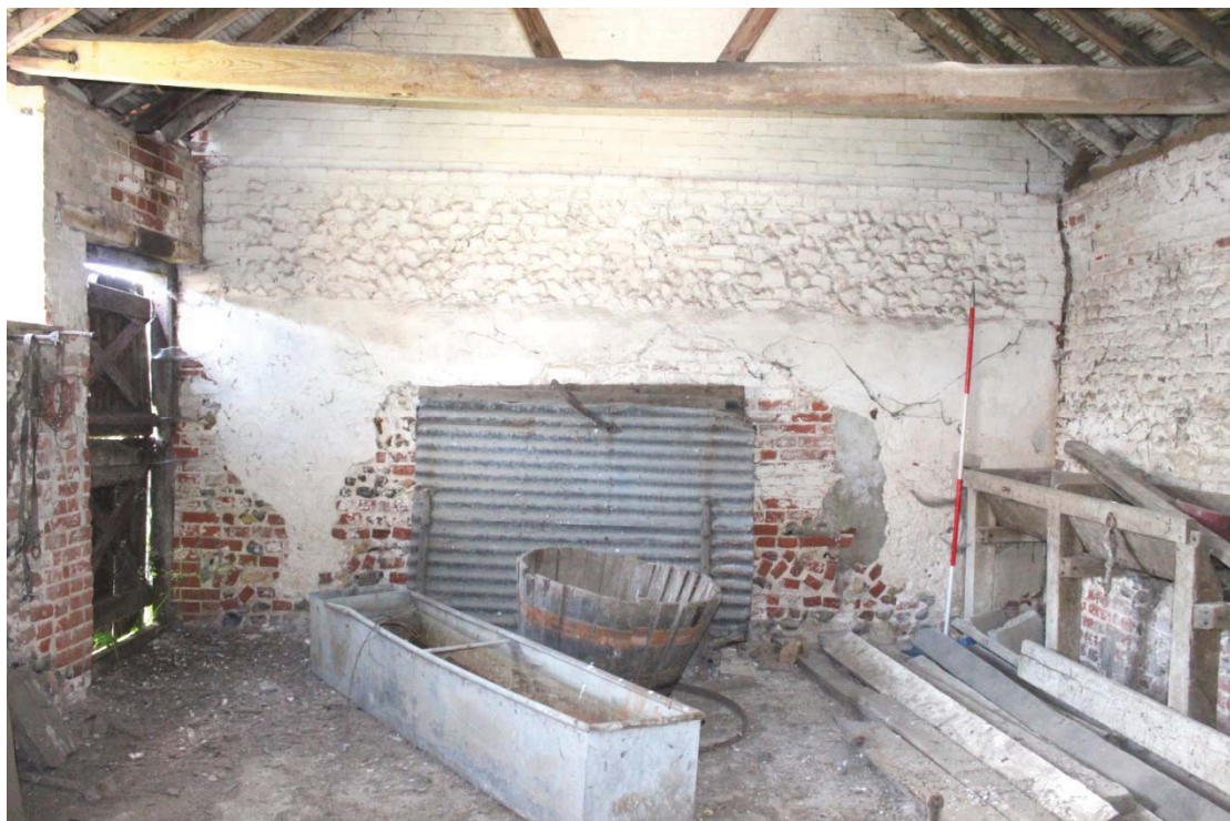
Illus. 8. Internal southern gable of northern stable (9) of Barn 1 showing its yard door to the left and an original boarded manger to right. Circular apotropaic marks are incised in the barn adjacent to the entrance and above the manger.
