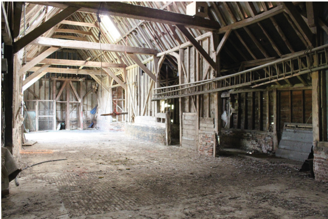
Illus. 12. Eastern interior of main barn (1) of Barn 2 showing the two original threshing bays B & E from left to right with an intact brick threshing floor in the foreground. The central doorway is a later insertion. The northern (left-hand) storey post of bay E to the right bears the carved date and initials shown in illus. 14.
