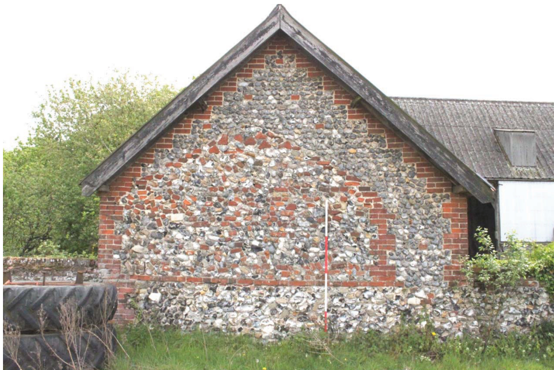
Illus. 16. Detail of western external gable of shed 3 of Barn 2 showing the outline of the narrower, earlier shed (as shown on the tithe map) which was incorporated into the present building.
