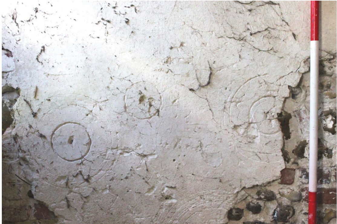
Illus. 9. Detail of circular apotropaic marks incised in lime render to eastern side of southern interior of stable (9) in Barn 1 (adjacent to entrance door to left).
