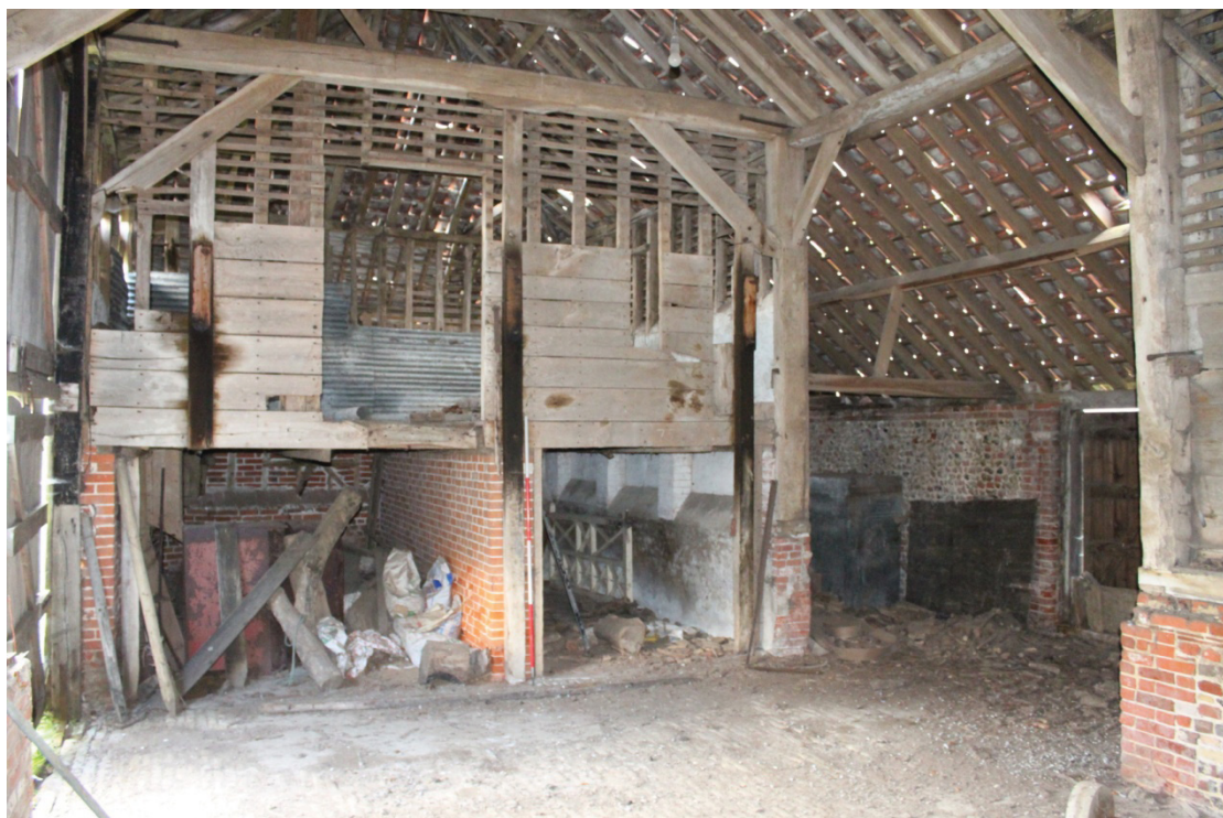
Illus. 4. Interior from west of main barn (1) of Barn 1 showing the early-20 th century inserted grain floor to the east of the central bay which retains an original brick threshing floor. The lean-to shed (1a) adjoining the yard is visible to the right. Note the unusually late straight braces to the tie-beams.
