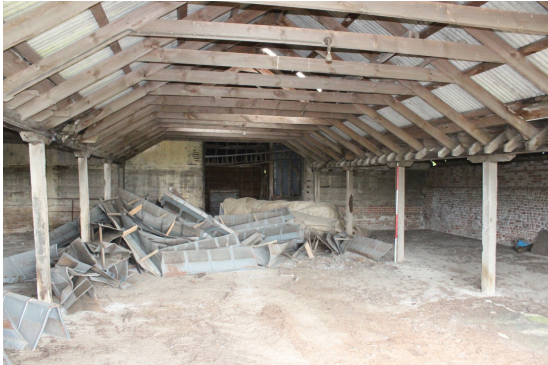
Illus. 15. Interior of 20th century covered cattle yard of Barn 2 from west showing open shelter-sheds 4 and 5 to left and right respectively. The southern entrance in bay E of the main barn (1) is visible in the rear, flanked by original two-tier cladding.
