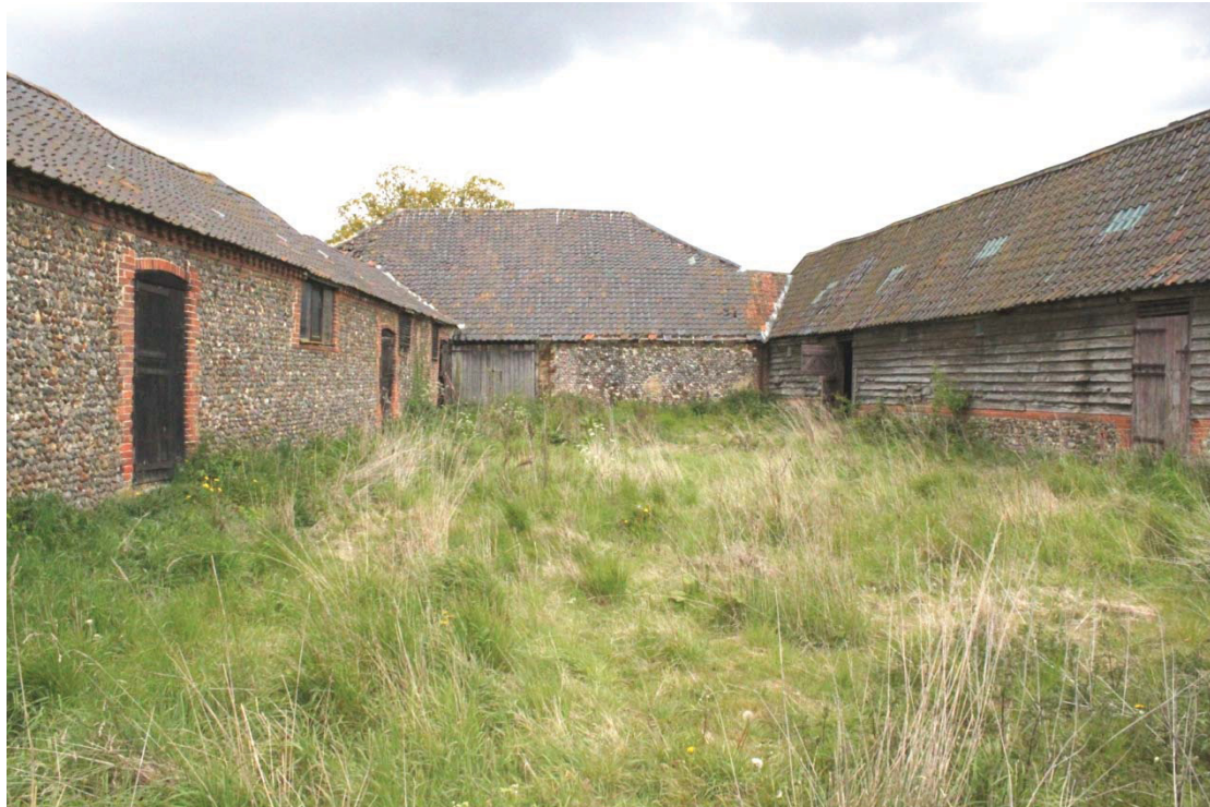
Illus. 3. Yard of Barn 1 from south showing hipped main barn (1) in centre with western stable range (7-9) to left and eastern cow-house range (3-5) to right. The latter was converted from an open-sided shelter shed.
