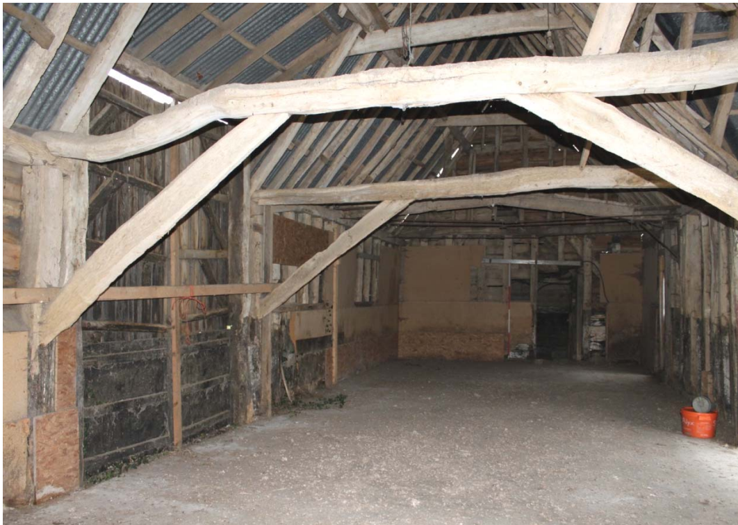
Illus. 4. Interior of main barn (1) from south showing the low arch-braces to the tie-beams flanking the entrance bay with roadside western doors to left. The north-eastern brace has been removed.
