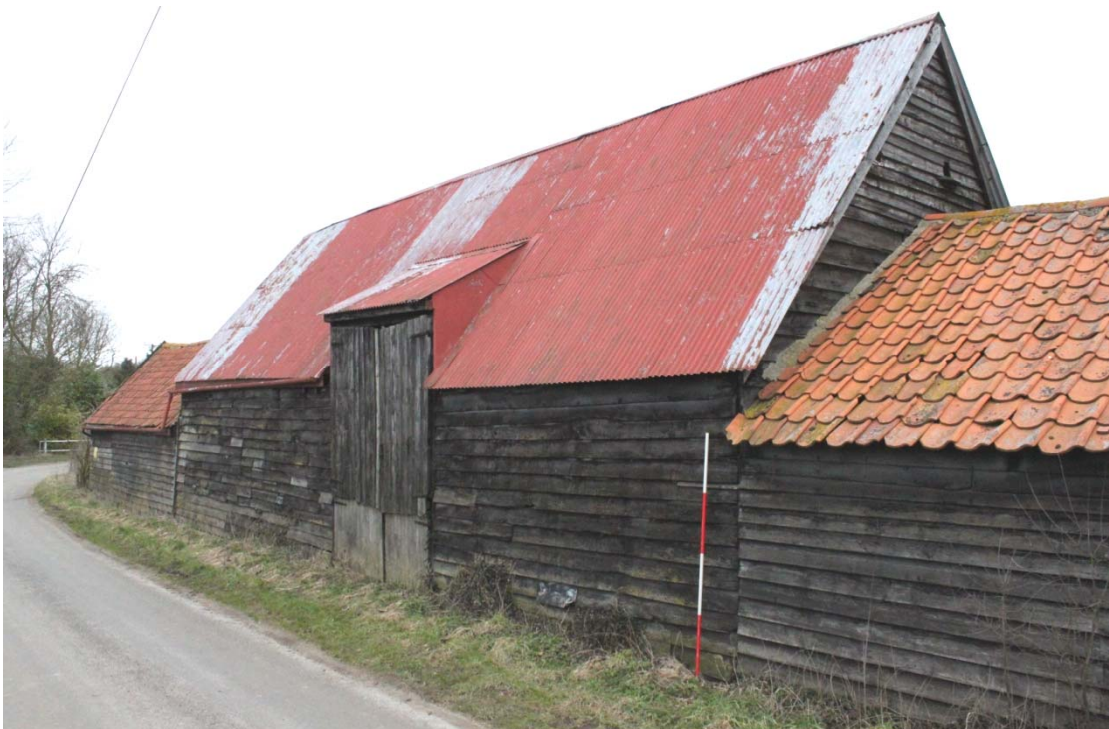
Illus. 2. Western exterior of barn (1) from Flowton Road to south-west showing pentice roof above entrance doors with pantiled sheds to left and right. The steep pitch of the barn's roof was designed for thatch but is now covered with corrugated iron.
