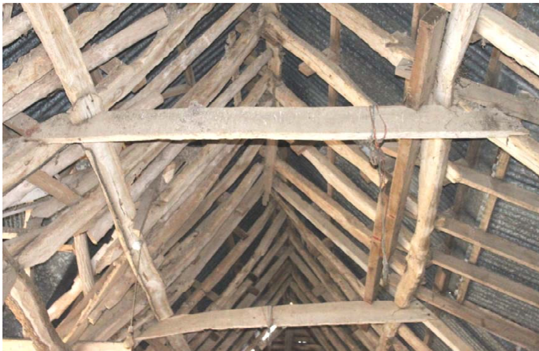
Illus. 10. Detail of roof structure from north showing nailed collars and clasped-purlins with the eastern porch to left and the softwood rafters of the 20 th century pentice roof above the roadside entrance to right.
