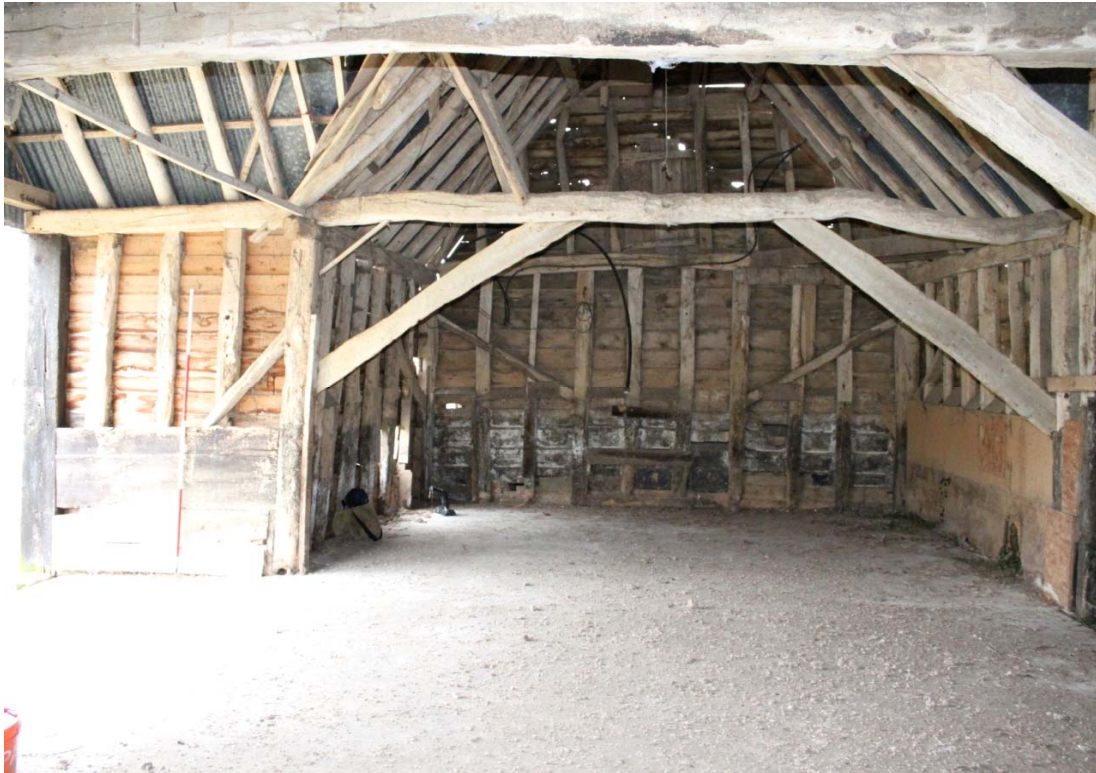
Illus. 9. Entrance bay of bay from north showing tie-beam of open truss continuing to form roof-plate of eastern porch to left. The straight primary bracing of the southern gable in rear contrasts with the earlier trenced bracing of the northern gable.
