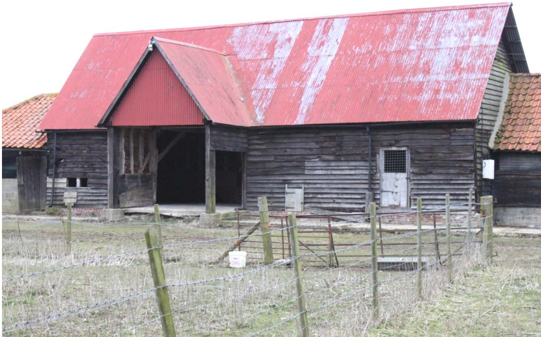
Illus. 3. Exterior of main barn (1) showing original gabled porch of penultimate southern bay to left and site of demolished lean-to shed against eastern elevation to right.
