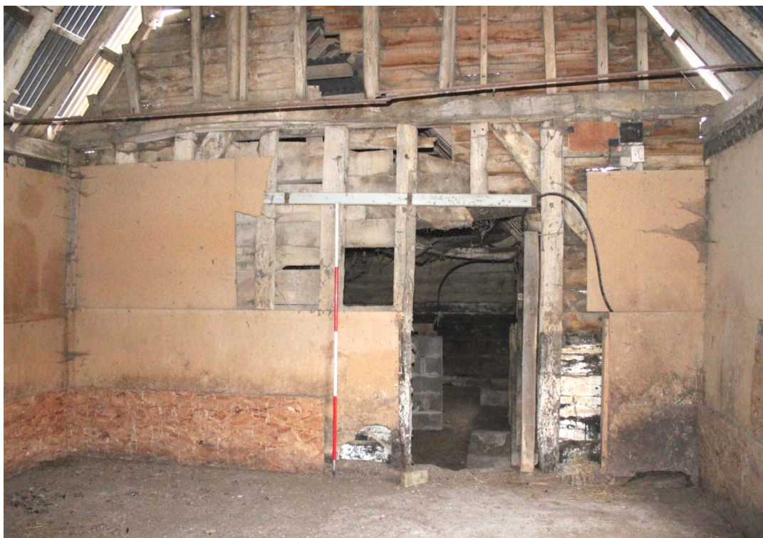
Illus. 5. Internal northern gable of barn showing original externally trenched braces behind modern boarding to right and left with door to cow shed (2). This gable is all that survives in situ of the early- to mid-17 th century barn on the site
