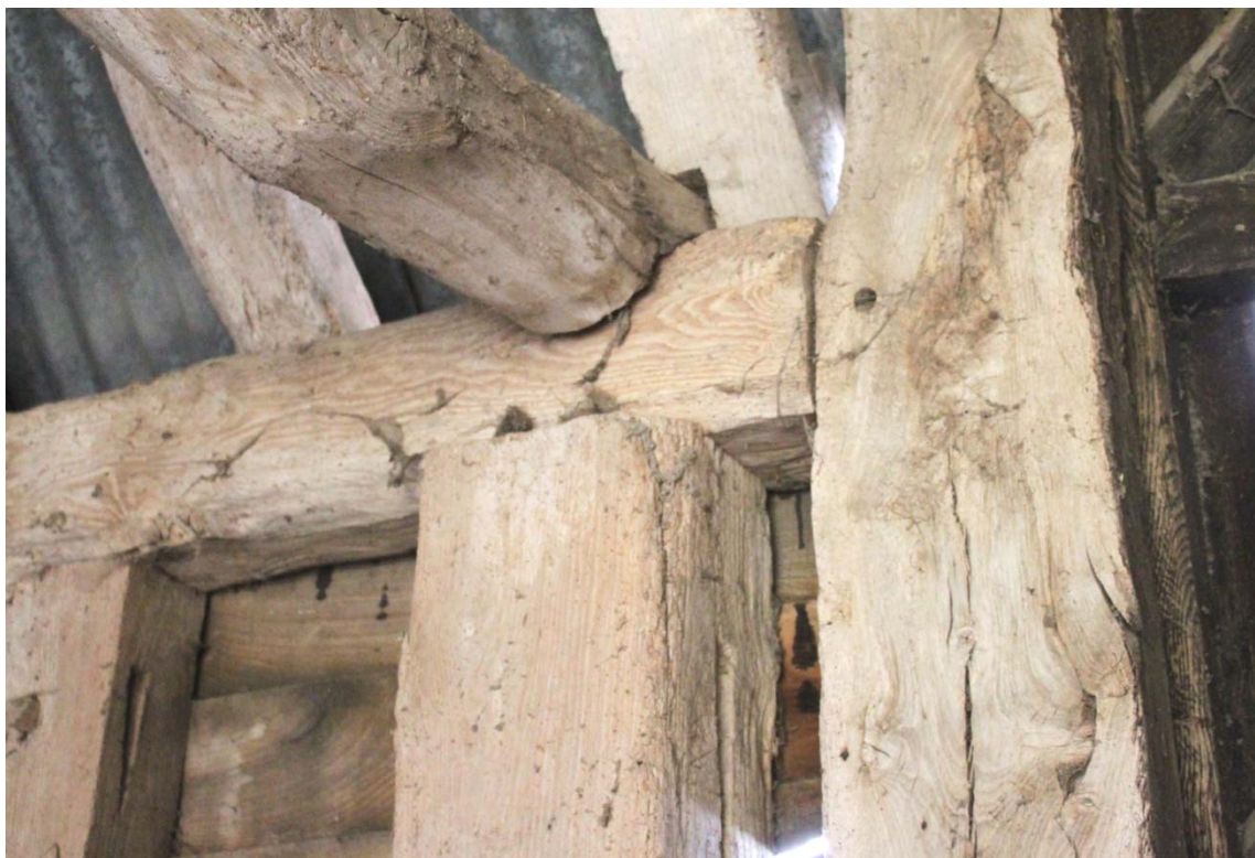
Illus. 8. Detail of un-jowled storey post to south of western entrance and roof-plate tenoned to door jamb.
