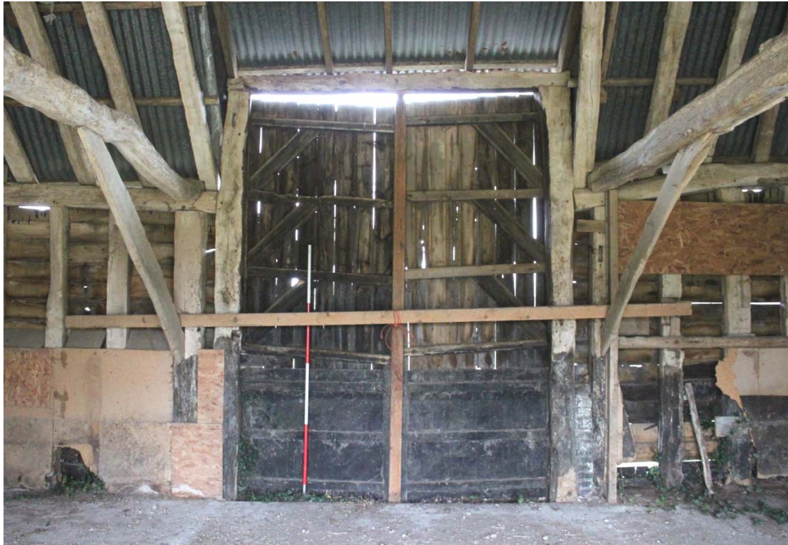
Illus. 7. Western interior of penultimate southern bay showing half-hung roadside entrance doors interrupting roof-plates with un-jowled but arch-braced storey posts to left and right. This entrance may have formerly possessed a vertical gable. The floor is of modern concrete with no trace of a threshing floor
