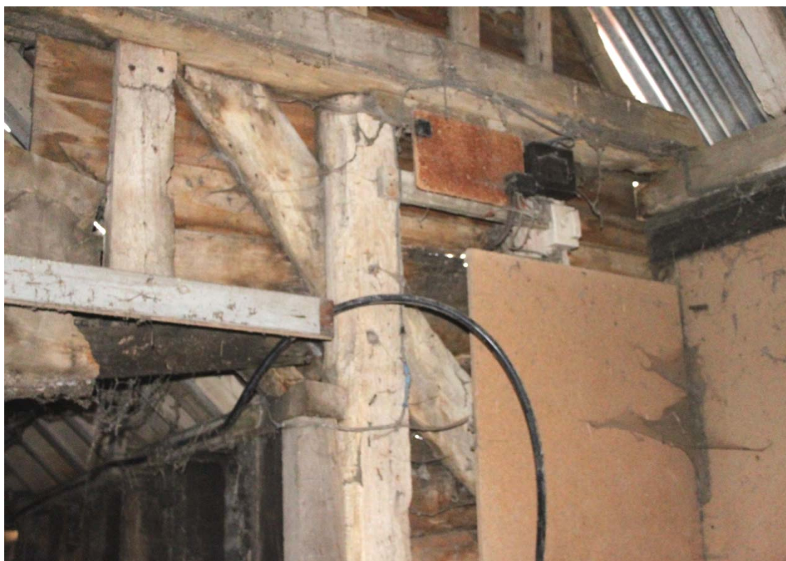
Illus. 6. Detail of externally trenched 17 th century brace in north-eastern corner of barn, showing door to cow-shed (2) adjoining northern gable to left.
