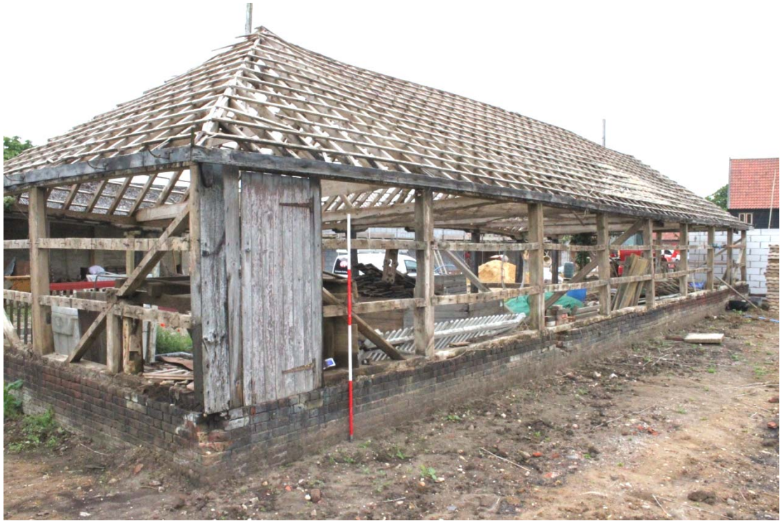
Illus. 5. Western exterior from north-west showing northern gable and door to left (re-used as cladding) with post-and-rail construction fully exposed. The converted barn is visible to the right.
