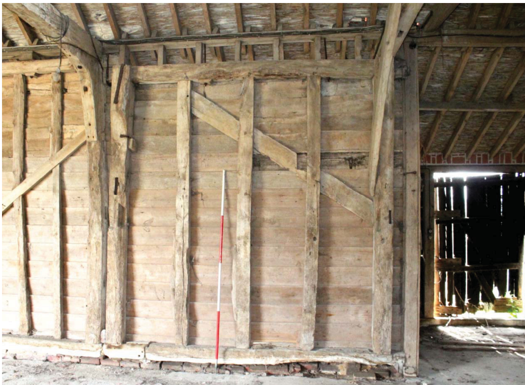
Illus. 8. Southern interior of single 17th century bay (1) showing 19th century bay to left (3) and rebuilt entrance bay with lean-to porch of 3-bay barn (2b) right. Note the externally trenched 17 th century brace to the right and the primary brace interrupting the studs to the left.
