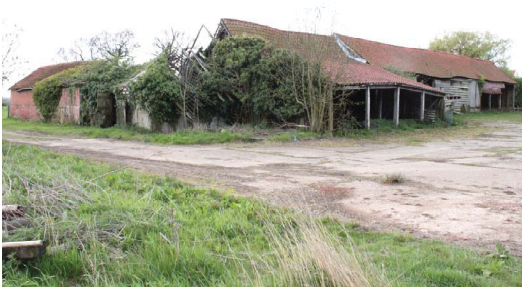
Illus. 3. Exterior of farm complex from north-east showing the partly collapsed early-19 th century granary and stable range (4 & 5) to the left of the barn. Its steeply-pitched roof structure was probably designed for thatch and is the earliest to survive on the site.
