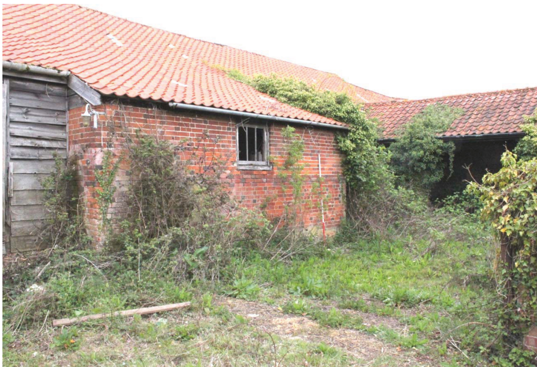
Illus. 14. Exterior of lean-to shed (10) from south-west showing the central shelter shed (9) in rear to right and the mid-19 th century lean-to porch of the 17 th century entrance (2b) to left.
