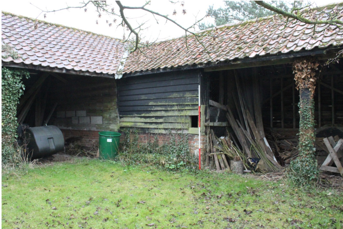
Illus. 5. Exterior from north-west showing the junction of the two integral wings with the open shelter-sheds (1b & 2a) to left and right respectively and the enclosed loose box or feed store (2b) in the centre.
