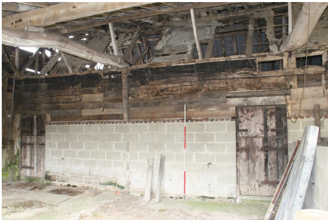
Illus. 8. Northern end of western exterior of stable (2) from adjoining open shed (4) showing lower walls of 20 th century cement blocks and the doors to the northern and central internal compartments to left and right respectively.
