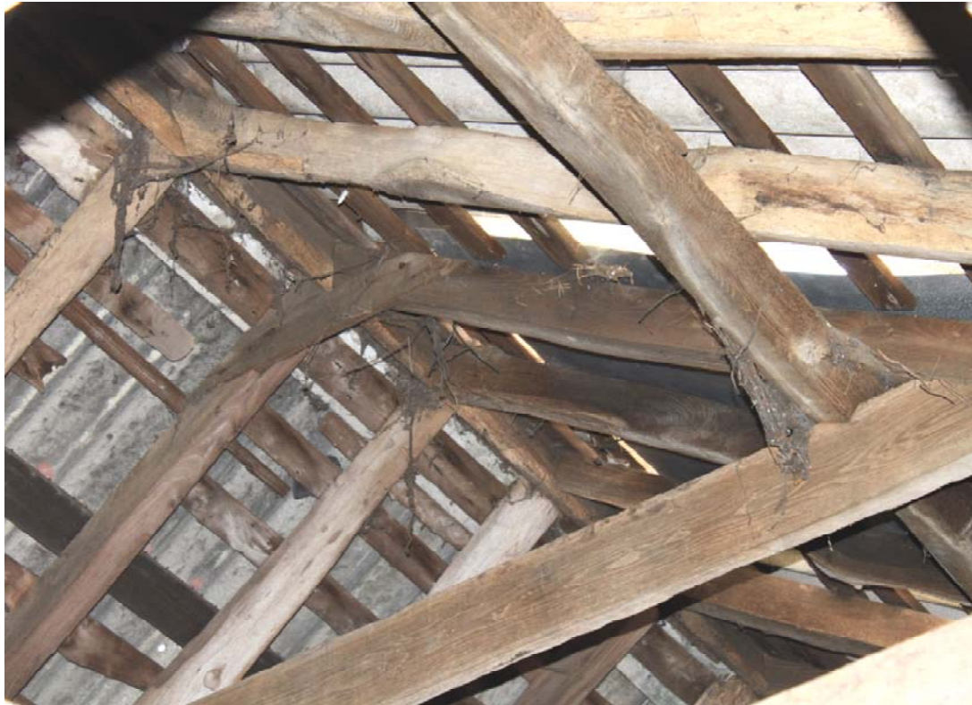
Illus. 8. Detail of nailed softwood roof structure of coach house (1) above modern ceiling.
