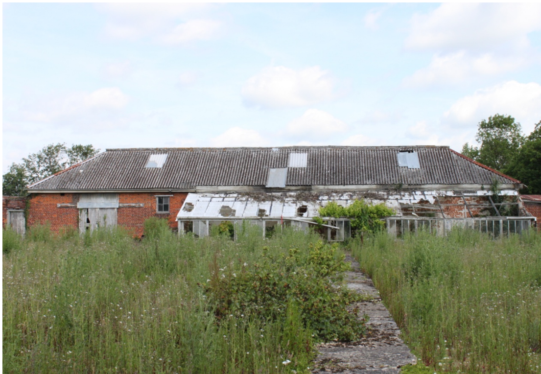
Illus. 2. Southern exterior of coach house from walled garden showing hipped roof of corrugated asbestos with conservatory to right and inserted sliding door to left.
