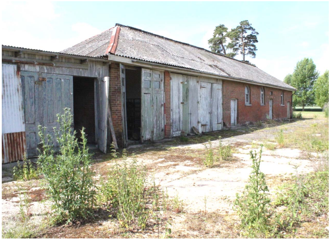
Illus. 4. Exterior from north-east showing northern facade with doors to vehicle sheds (2 & 3) to left with 20 th century lean-to shed (4) to extreme left.
