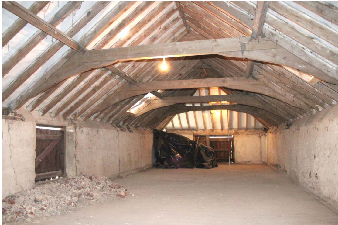
Illus. 9. Southern granary loft seen from north and showing loading doors to the left and in the southern gable with the replacement clasped-purlin softwood roof structure of the late-19 th century.
