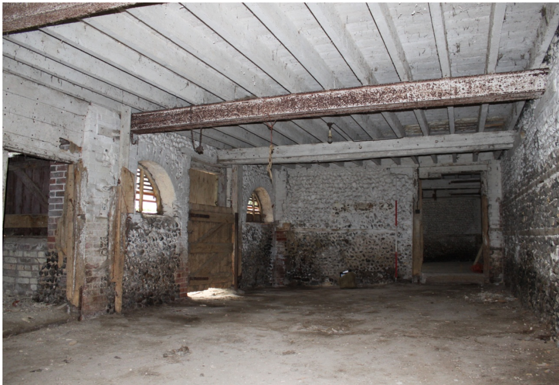
Illus. 6. Interior of northern stable (1c) from north showing southern entrance to left and secondary door to central stable (1b) right. The boarded partition of the narrow chaff box is visible to the left and the ceiling is a late-19 th century replacement.
