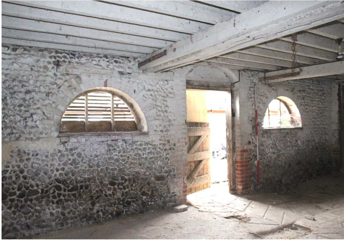
Illus. 7. Internal eastern elevation of the central stable (1b) showing the central entrance flanked by arched windows.
