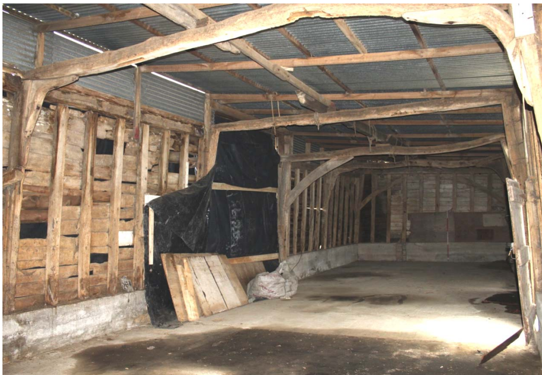
Illus. 12. Interior of the early-17 th century five-bay threshing barn (4) from east showing southern elevation to left with a single original tie-beam arch-brace extant and a modern single-pitch roof.
