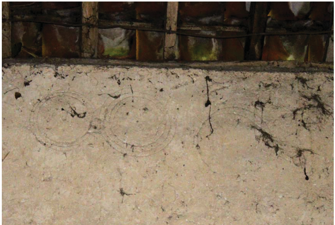
A2.8 Detail of incised concentric apotropaic circles at the eastern end of the northern internal elevation, showing pantiles and rafters above.
