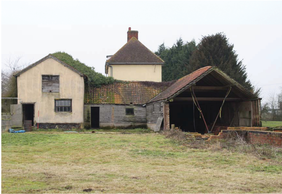
A2.3 General view from site of demolished barn to east showing clay-lump stable (1) to left with farmhouse (4) and enclosed 20 th century shelter shed (3) in centre. The brick plinth of the demolished 20 th century animal shed (3) is visible to right. The ground-floor door and window of the stable are secondary but the hay loft door above is original.
