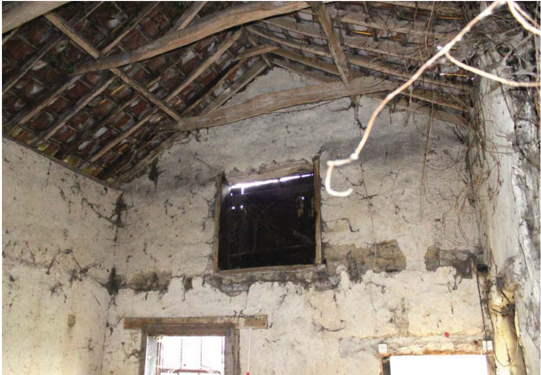
A2.7 Interior of eastern gable showing original loft door scars of removed ceiling joists. Groups of circular apotropaic marks have been incised into the internal daub to the left and right of the door and to the northern elevation visible to the left (see A2.8 below). Similar marks lie to the east of the loft window in the southern elevation (top-right).
