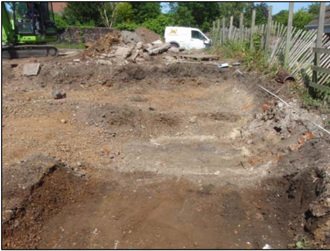
Plate 1. Cottage foundations 0014 (facing northeast)
