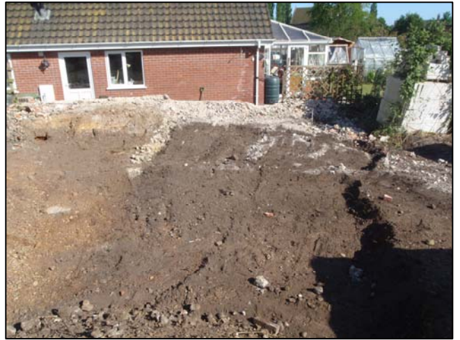
Plate 2. Possible terrace and shed foundation 0031 (facing southeast)
