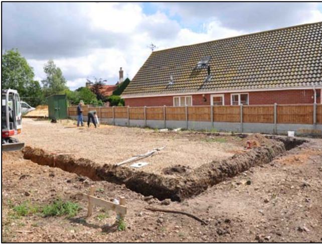
Plate 7. General view of foundation (facing east)
