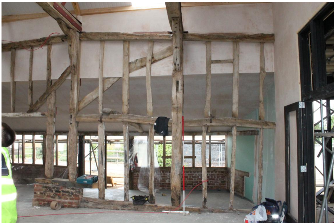
Illus. 6. Western bays of northern interior of eastern barn (1b) showing an original trenched corner brace with the position of its missing western gable to left.
