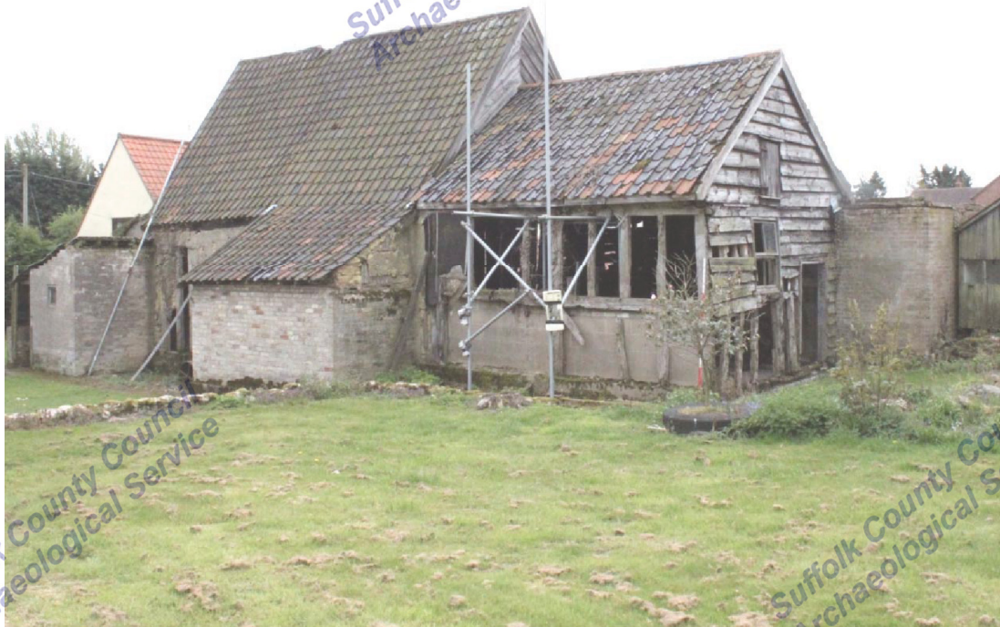
Illus. 4. Exterior of barn from north-west showing the low roof of the rebuilt western end to right and the formerly thatched steeply pitched 17 th century roof of the central and eastern bays to left.
