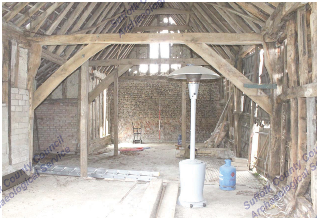
Illus. 6. Interior of barn from west showing 17th century arch-braces to tie-beams of central bay
