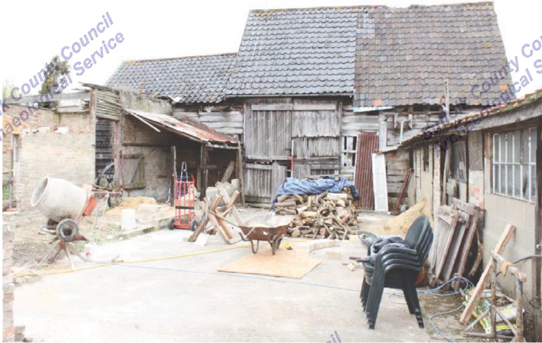
Illus. 5. Southern exterior of barn from cattle yard showing raised roof over central entrance doors and rebuilt western end to left.
