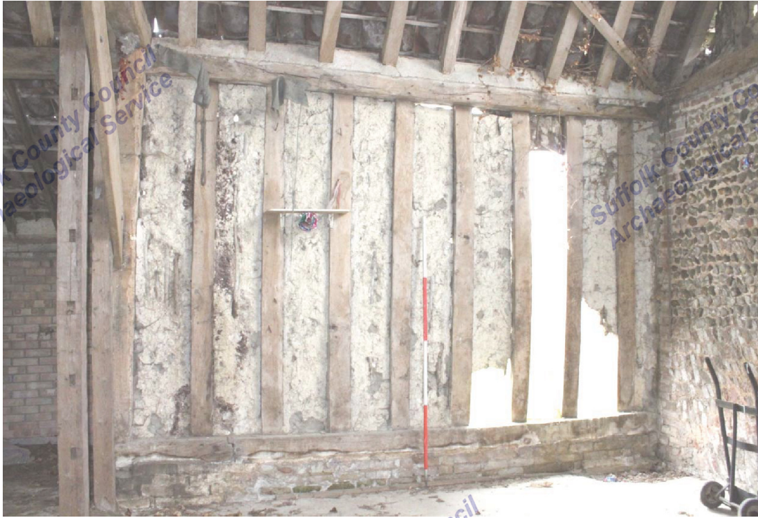
Illus. 9. Northern interior of eastern bay showing good-quality 17 th century studs with externally trenched wall brace (top-right) and rebuilt 19 th century flint gable to right.
