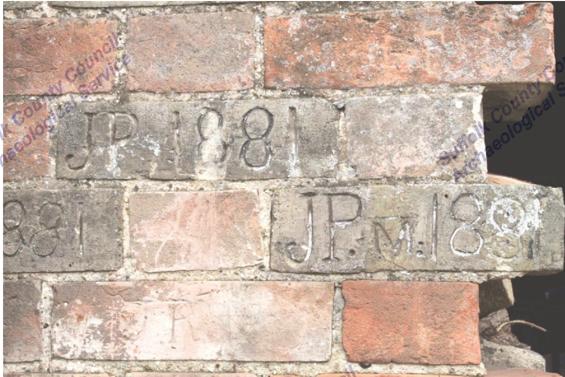
Illus. 13. Detail of the boldly incised initials and dates in the brickwork of the southern exterior of the eastern shed (3): 'J.P. 1881'. The shed is not shown on the Ordnance Survey of 1886 and the 'Woolpit white' bricks are probably re-used from an earlier building (they differ in colour from the surrounding red brickwork).
