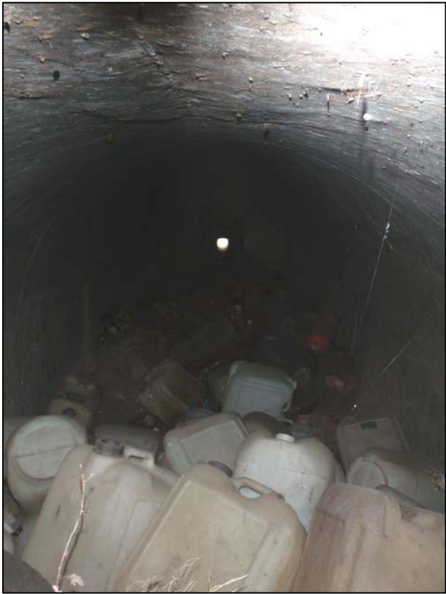
Plate XI. View from the manhole into the shelter, camera facing south-east
