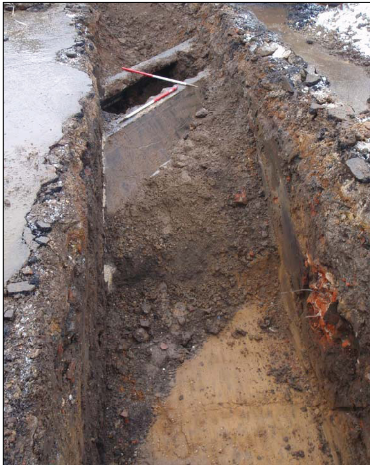
Plate VIII. Trench 4, air-raid shelter and cut, camera facing west
