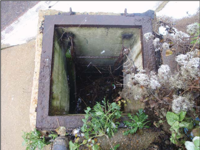
Plate X. View down manhole, camera facing north-west
