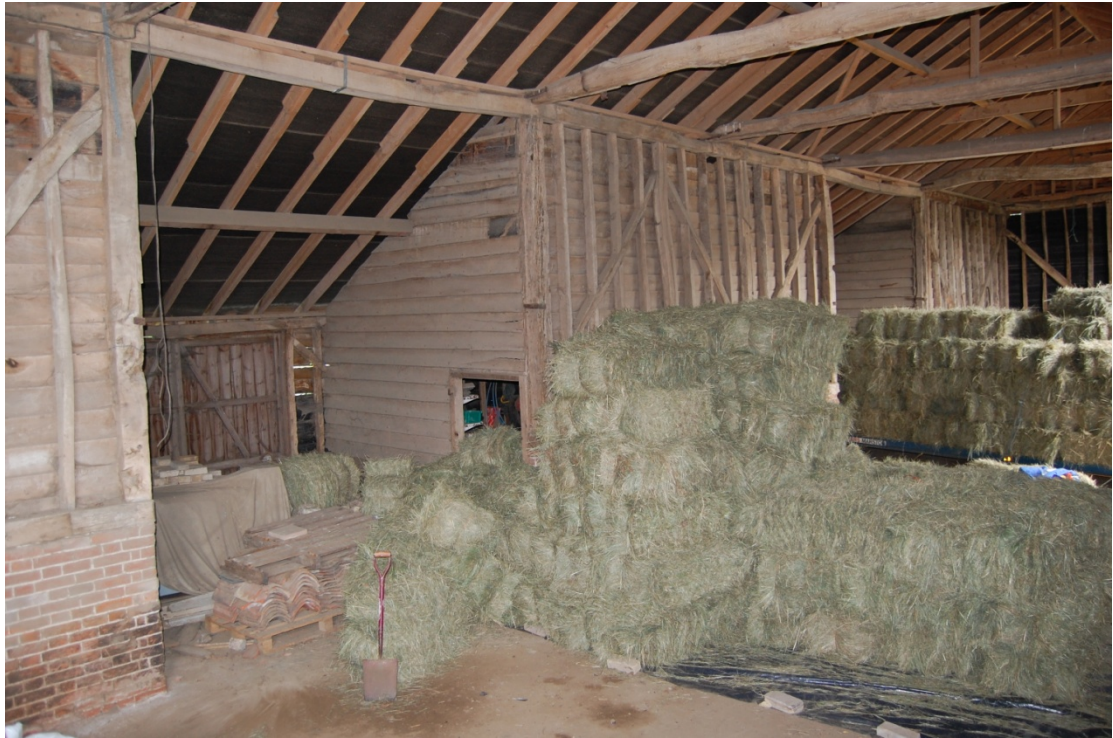
Illus. 7. Interior of the main barn showing the rear (eastern) doors of the two threshing bays linked by integral lean-to sheds. Note the recently renewed softwood roof structure.
