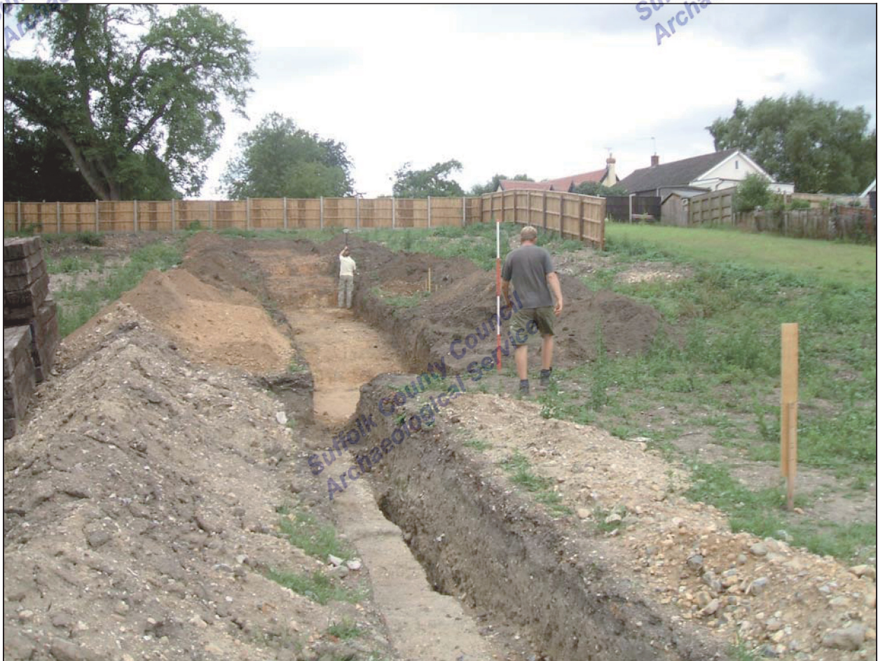
Plate 2. Terraced slope, looking south-south-west
